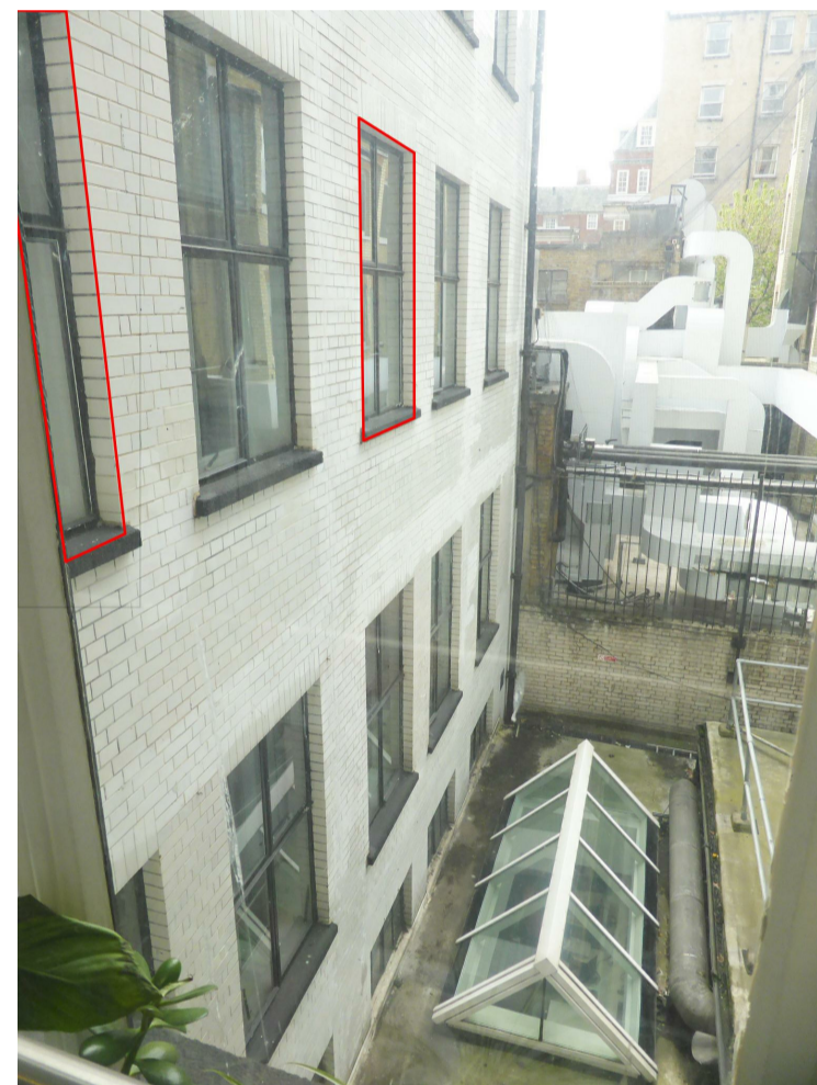
Photos (1) Existing elevation to the lightwell. Windows to be replaced by aluminium louvres indicated by red boundaries.
