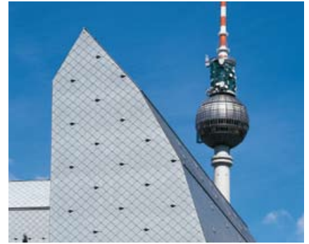
Head Offices of Berlinwasser Holding AG, Berlin, Germany
