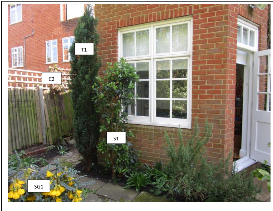
View of rear right corner
