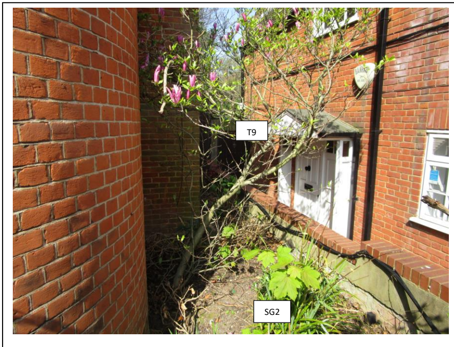
View of right front flank
