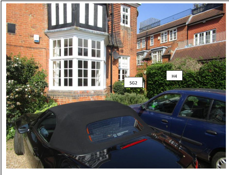
View of front right bay
