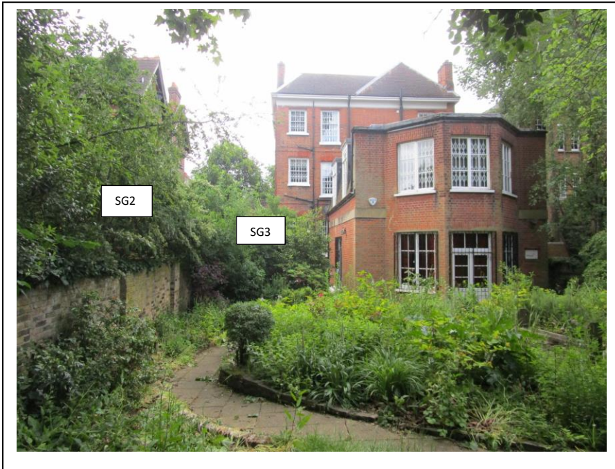
View of rear elevation
