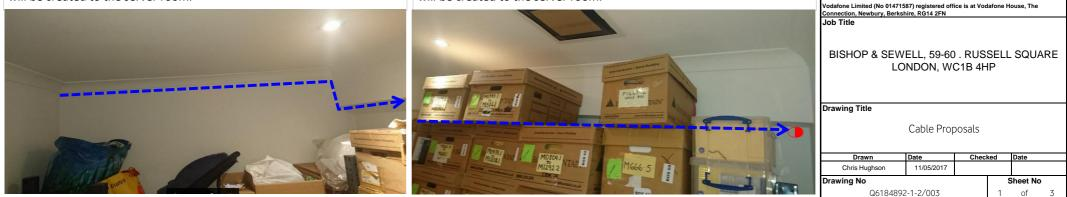
7. The fibre will be routed again with uPVC trunking to reach the cable tray, and then this route will be followed down and under the raised floor to the comms cabinet
