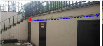
3. From here, 50mm uPVC trunking will be installed to route the fibre to the back wall of the office where another entry point will be created to the records room
