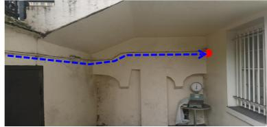
4. From here, 50mm uPVC trunking will be installed to route the fibre to the back wall of the office where another entry point will be created to the records room
