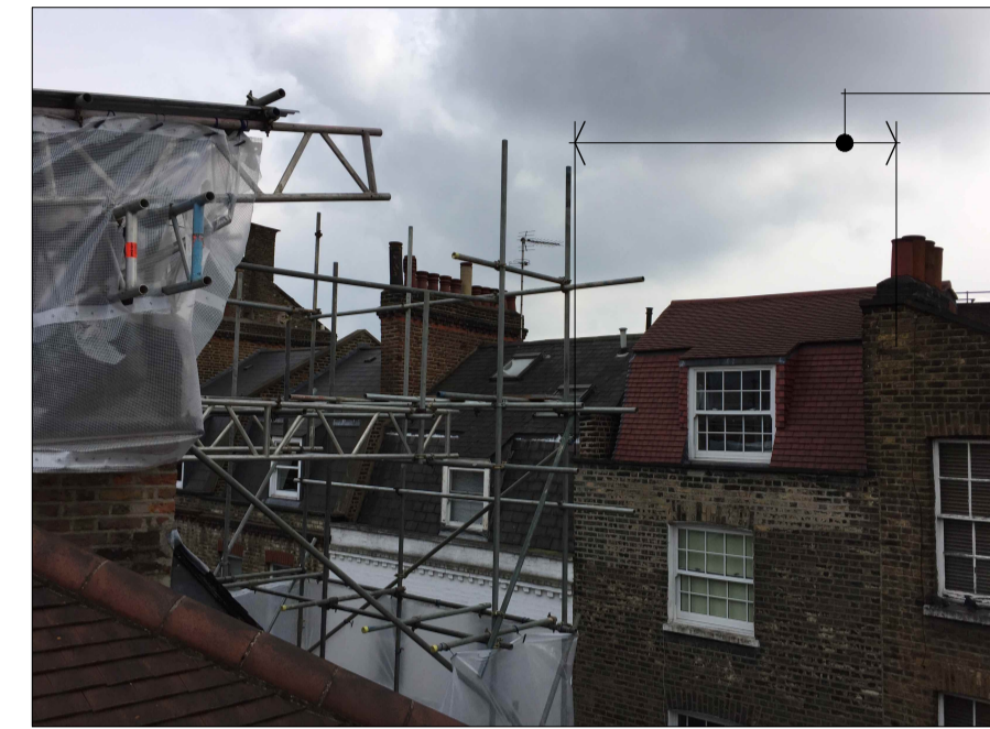
Flask Walk View at Roof Level
