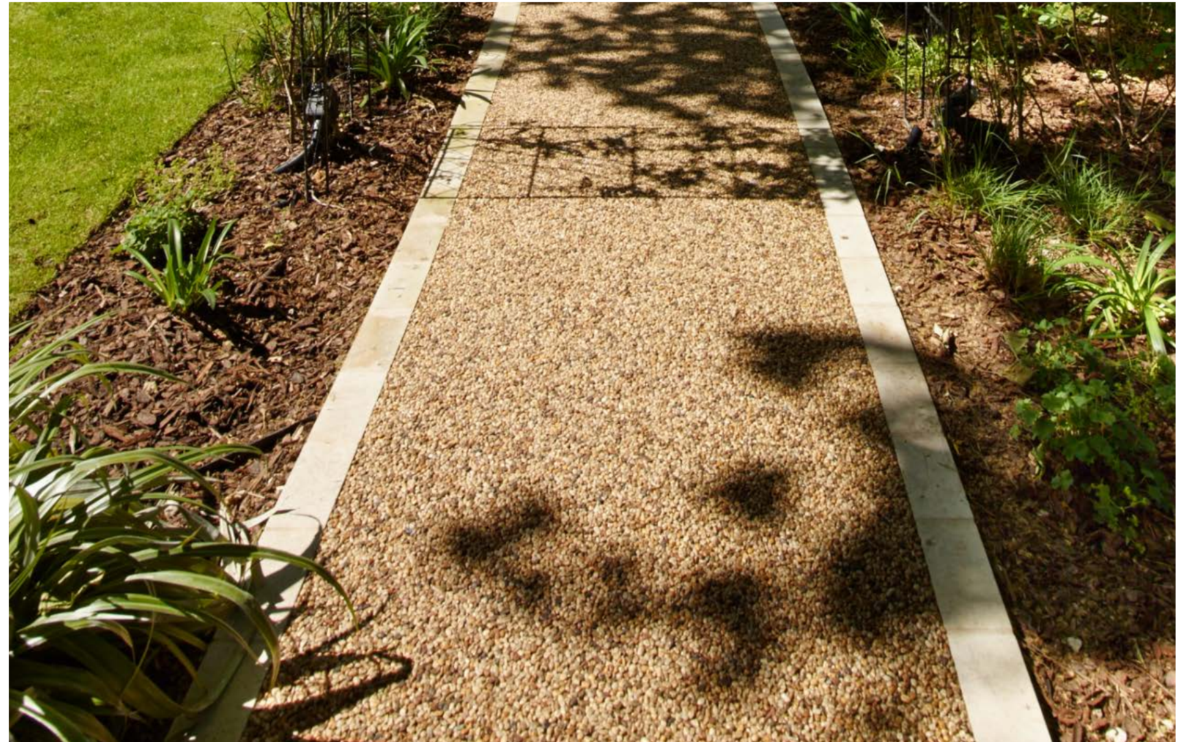
Permeable resin bound gravel footpath edged in stone OR a simple steel edge. To be used in rear footpaths and ramps
