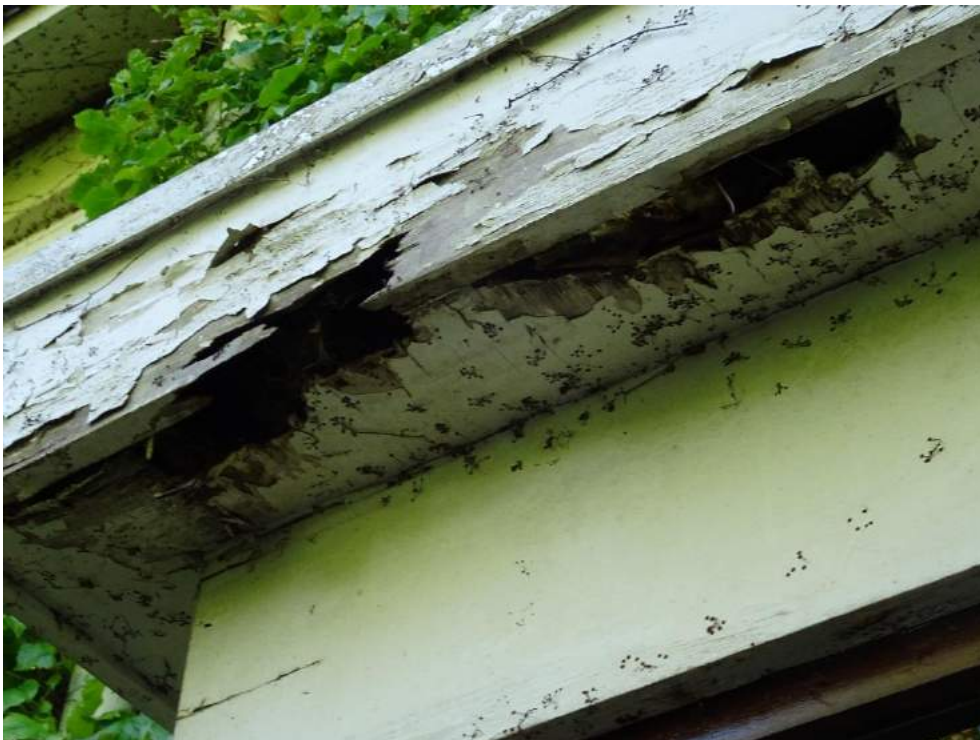
Photograph 10: Example of bat feature on Building 1
