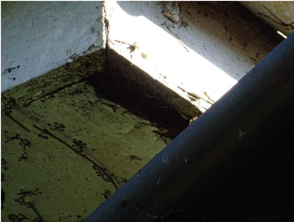
Photograph 9: example of bat feature on Building 1
