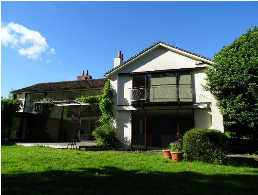
Photograph 7: Main House (Building 1)
