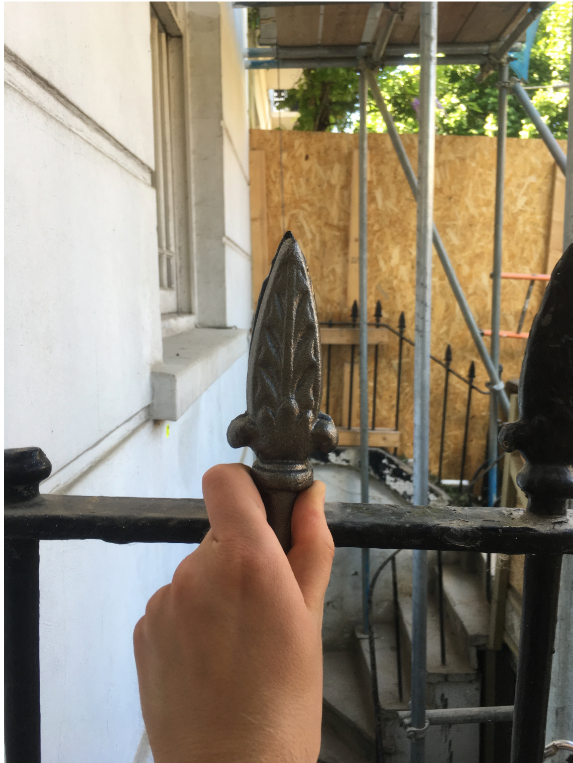
1 New railing head Infront of existing
