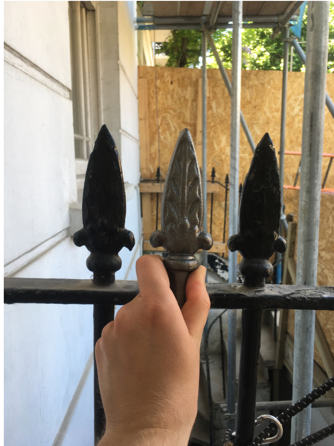
2 New railing head next to existing
