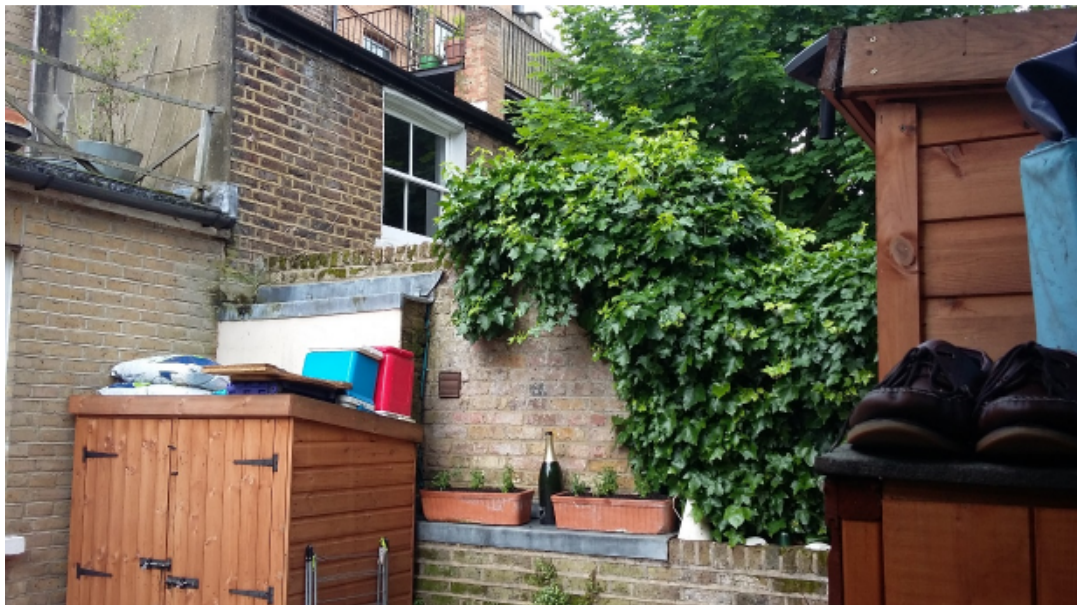
View to show edge of shed and edge of main building and other wooden structure (not part of this application)
