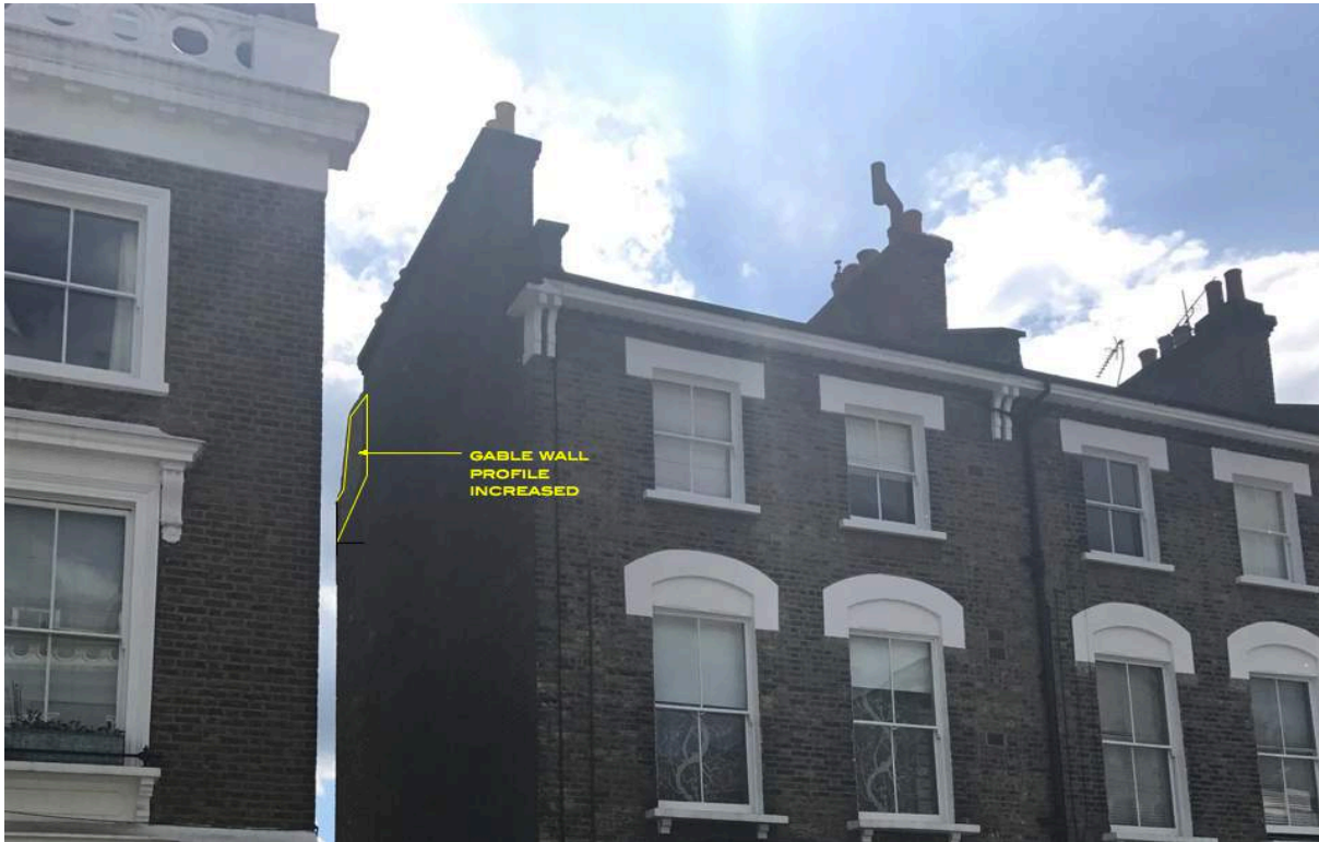
Image 7 - 31 Fitzroy Road – Gable Wall Profile Alteration
