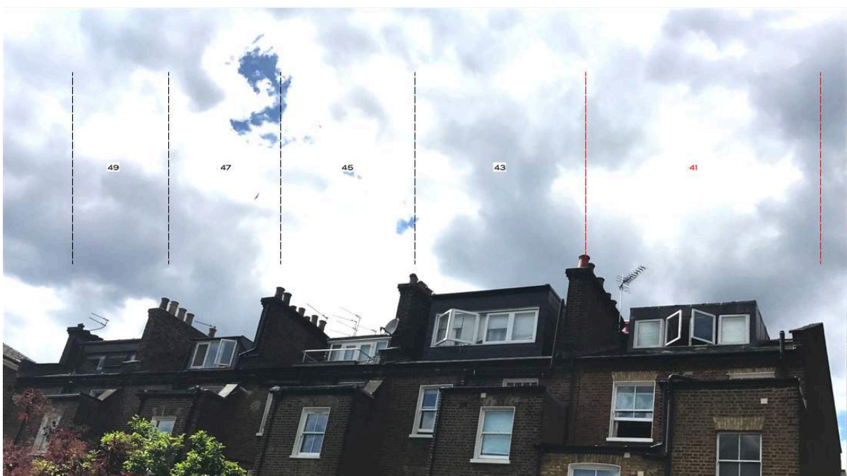
Image 6 – Rear Roof Extensions at 41 to 49 Fitzroy Road
