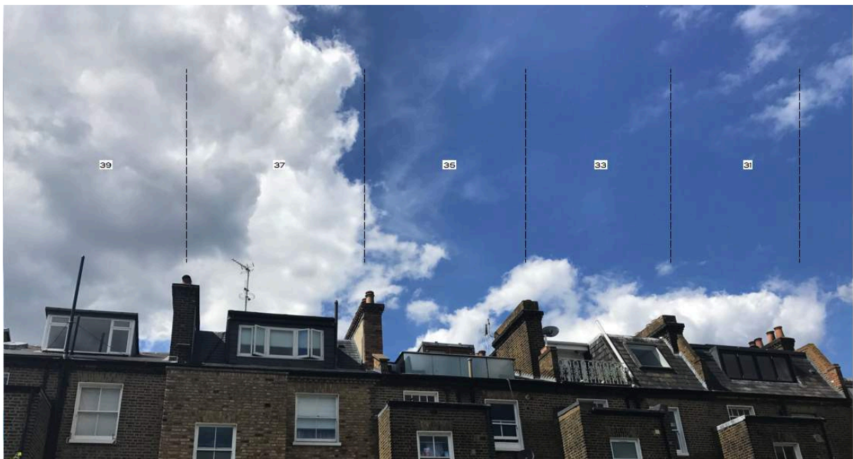
Image 5 – Rear Roof Extensions at 31 to 39 Fitzroy Road
