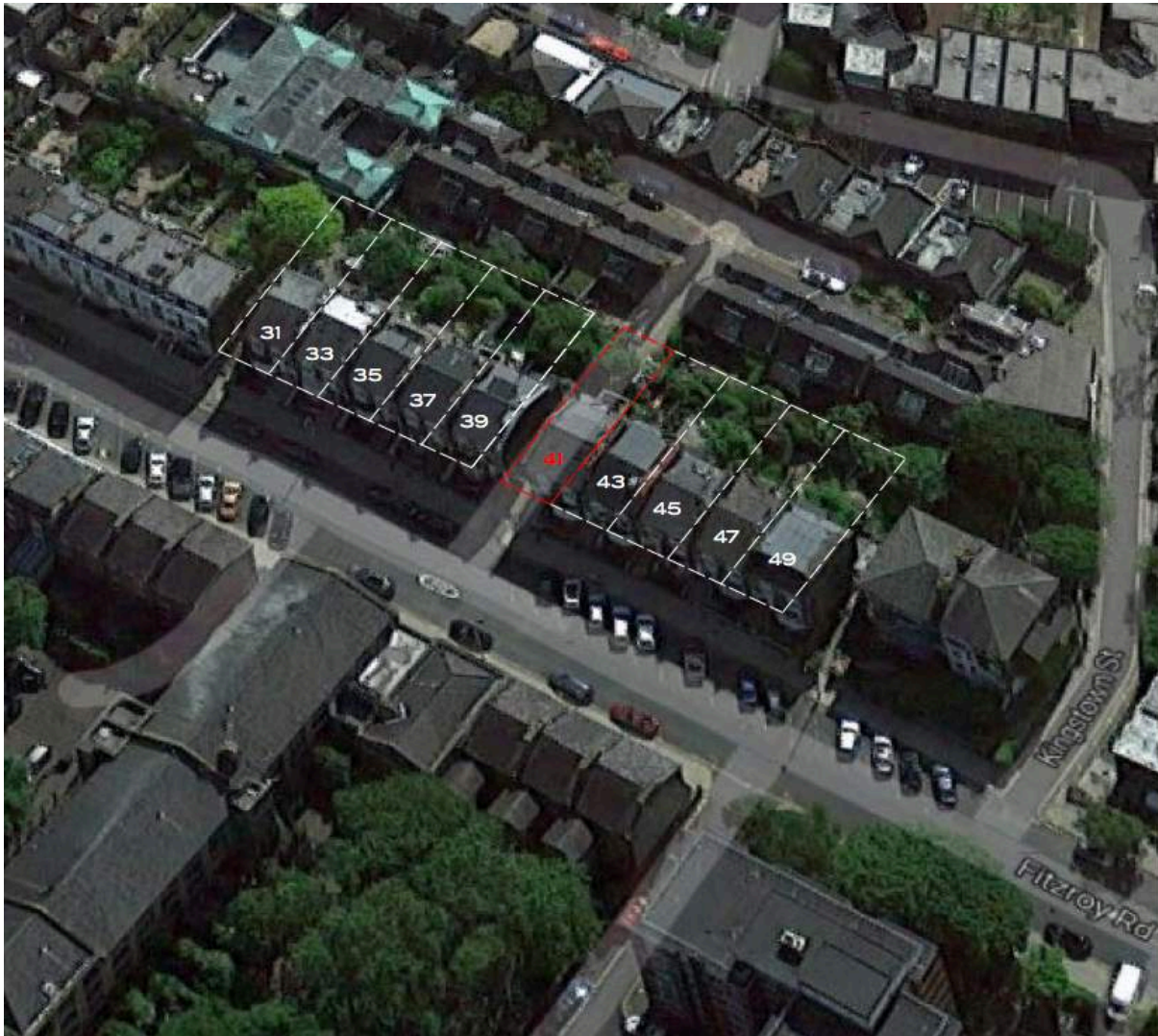
Image 1 - Aerial photograph showing 31 to 49 Fitzroy Road with the Application Property edged in Red
