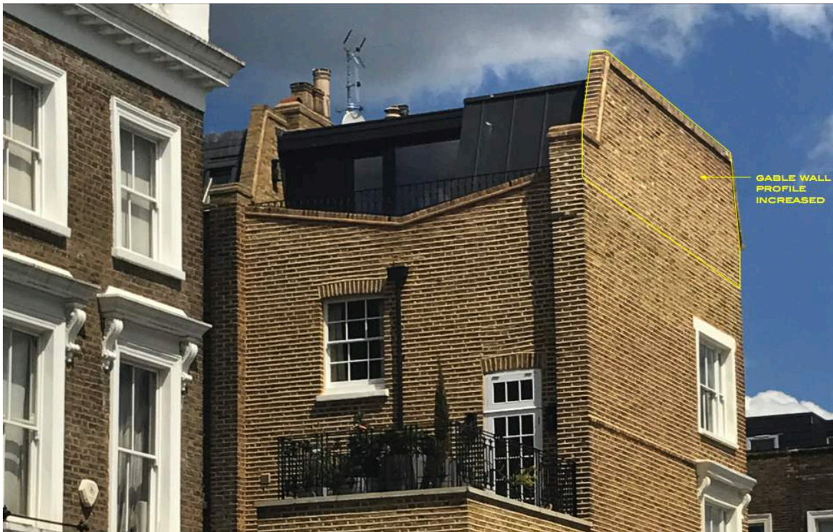
Image 8 - 38 Chalcot Road – Gable Wall Profile Alteration
