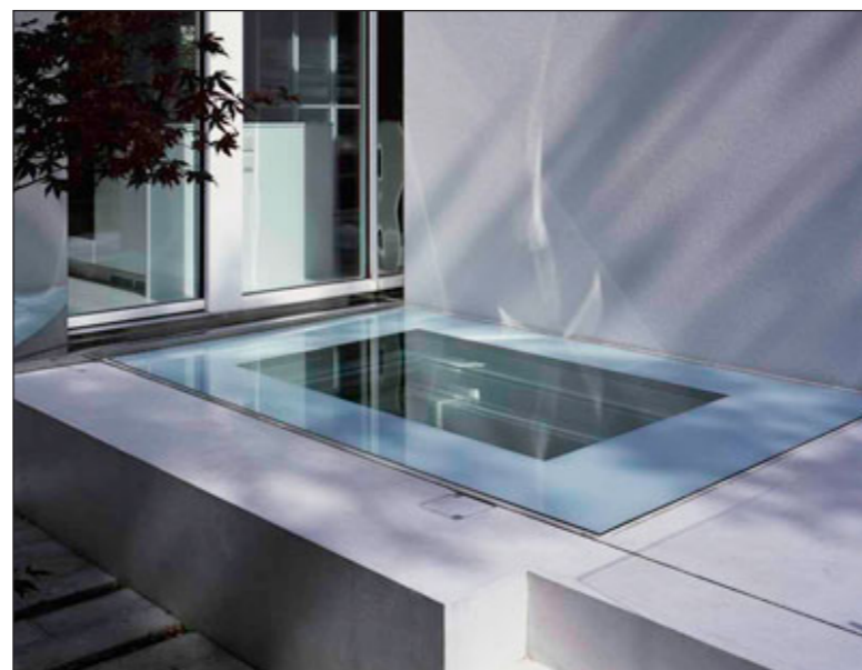
GLASS FLOOR ALLOWS LIGHT TO SPILL INTO THE LOWER GROUND FLOOR
