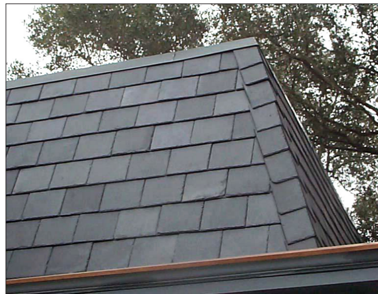
SLATE TILE ROOF FINISH FOR MANSARD ROOF
