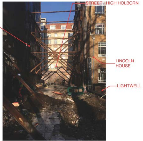
Basement at rear of site
