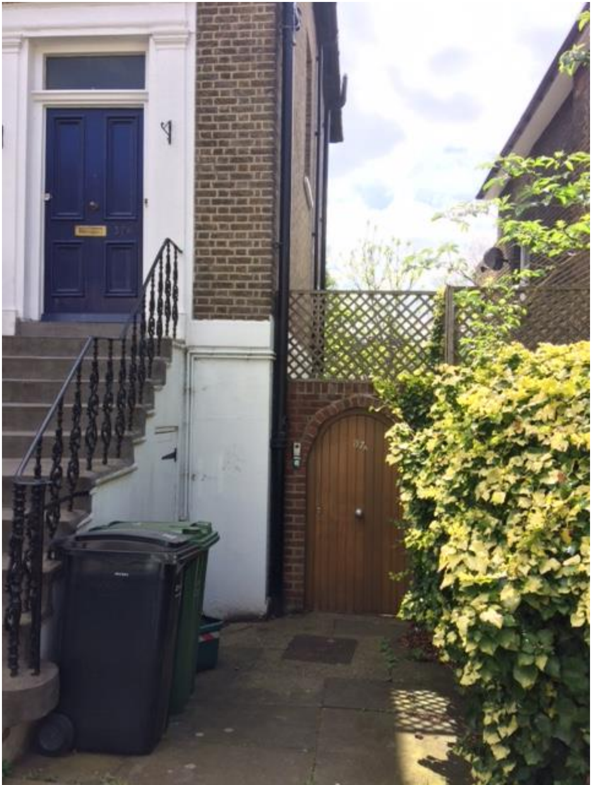
Photo 6 - Front of Property
