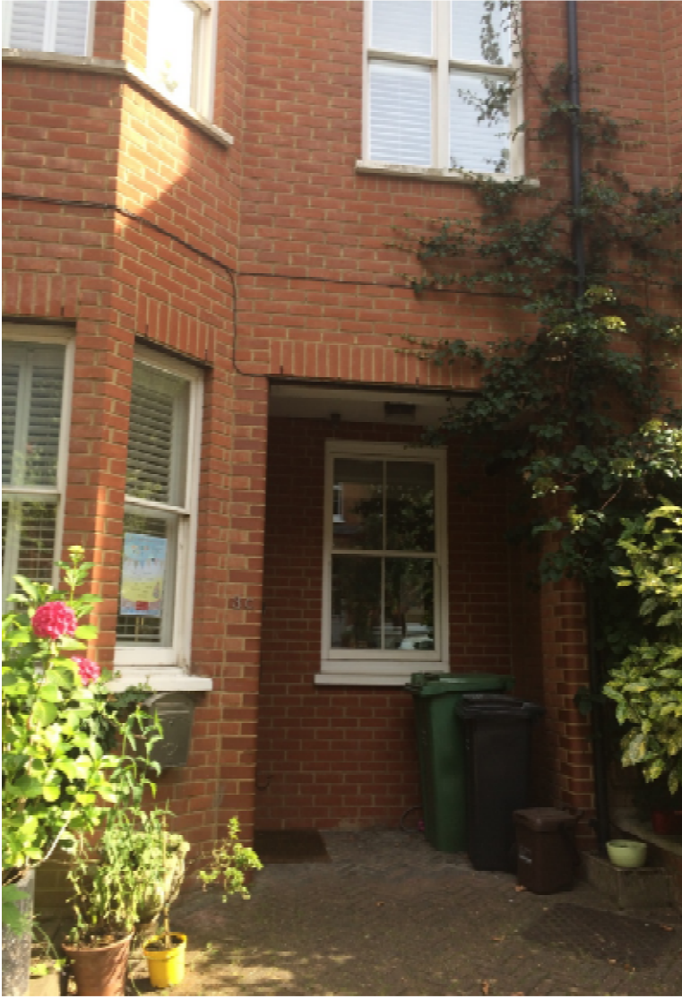
3. Existing front entrance of 3C
