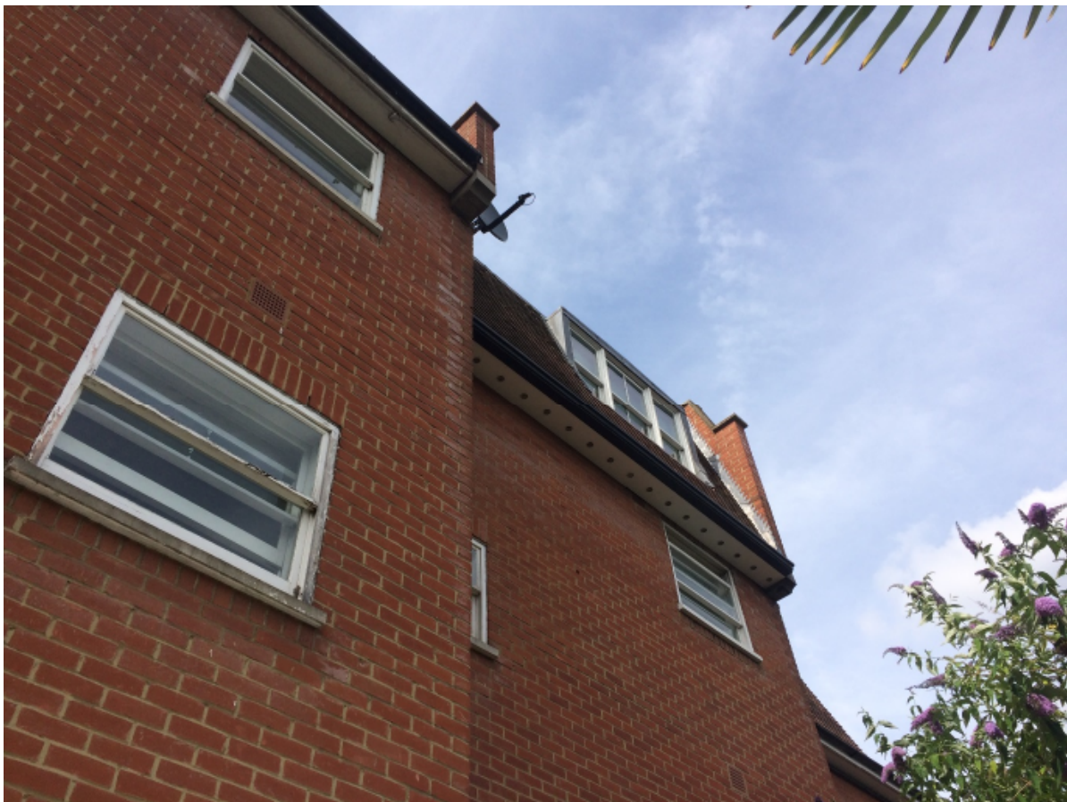
2. 3B Heath Hurst Road – rear roof extension
