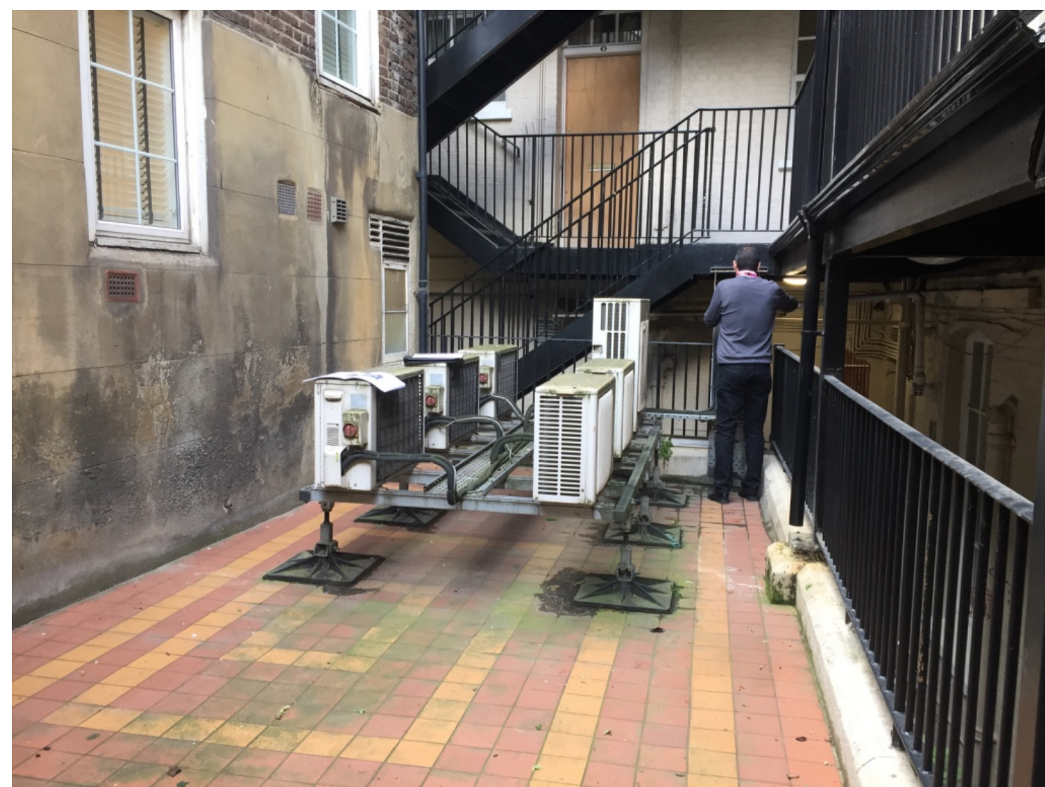
PHOTO OF EXISTING PLANT AREA
