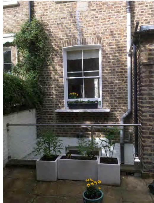
Rear elevation- kitchen window
