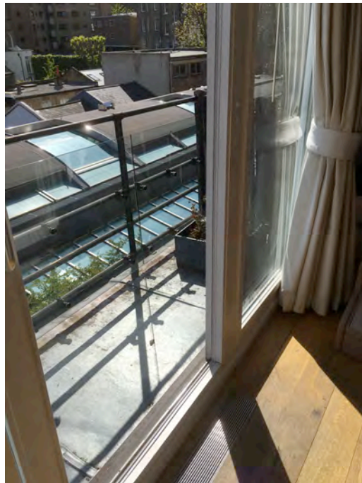
Third floor- rear elevation balcony and balustrade
