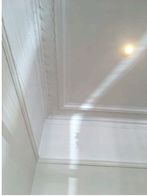
Ground floor- cornice to dining
