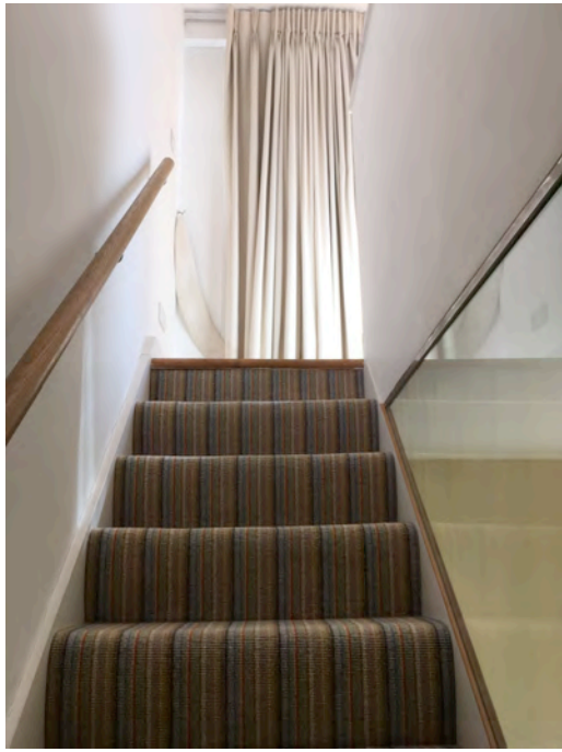
Second/ third floor- stair balustrade
