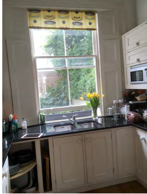
Ground floor- kitchen window
