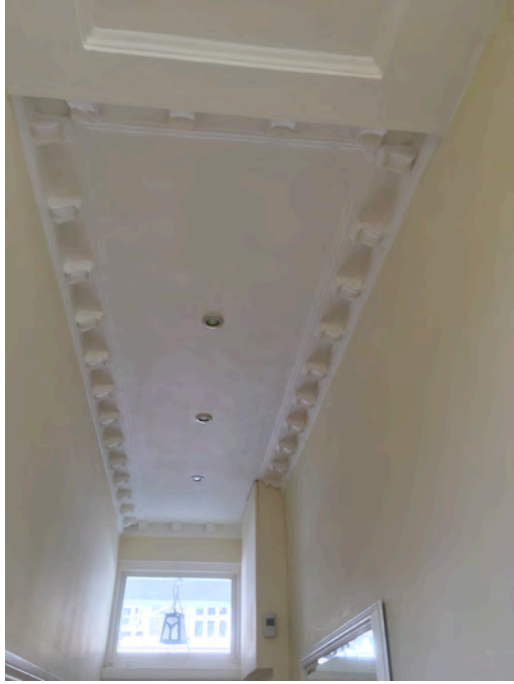
Ground floor- cornice to hall
