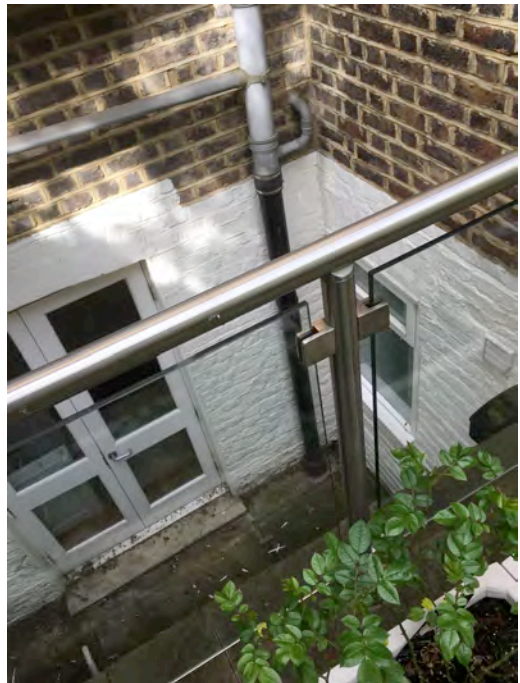
Rear elevation- rear light well- rear door and window
