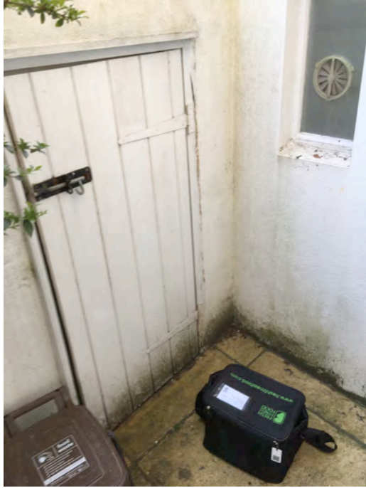
Front light well- existing vault door
