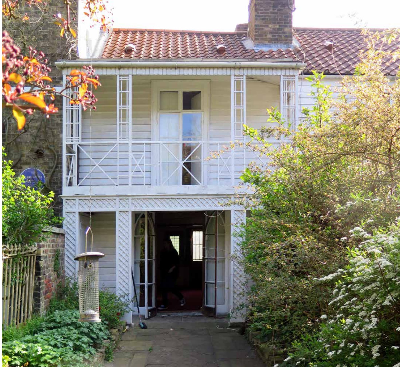
Existing west facing elevation (formerly the front)
