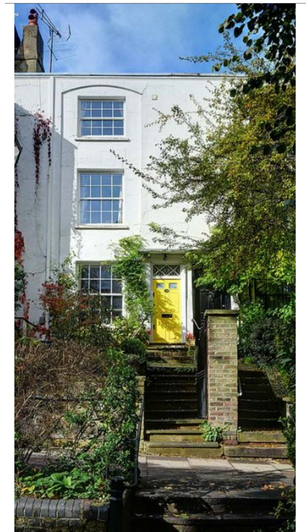
05. PHOTO OF FRONT ELEVATION - Showing Windows To Receive New Sashes
