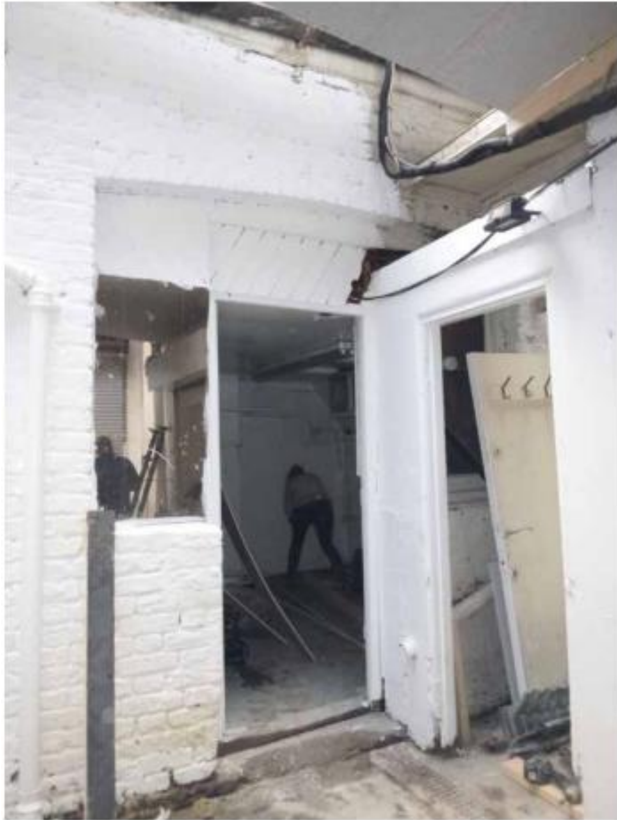
Above: Rear workshop building
