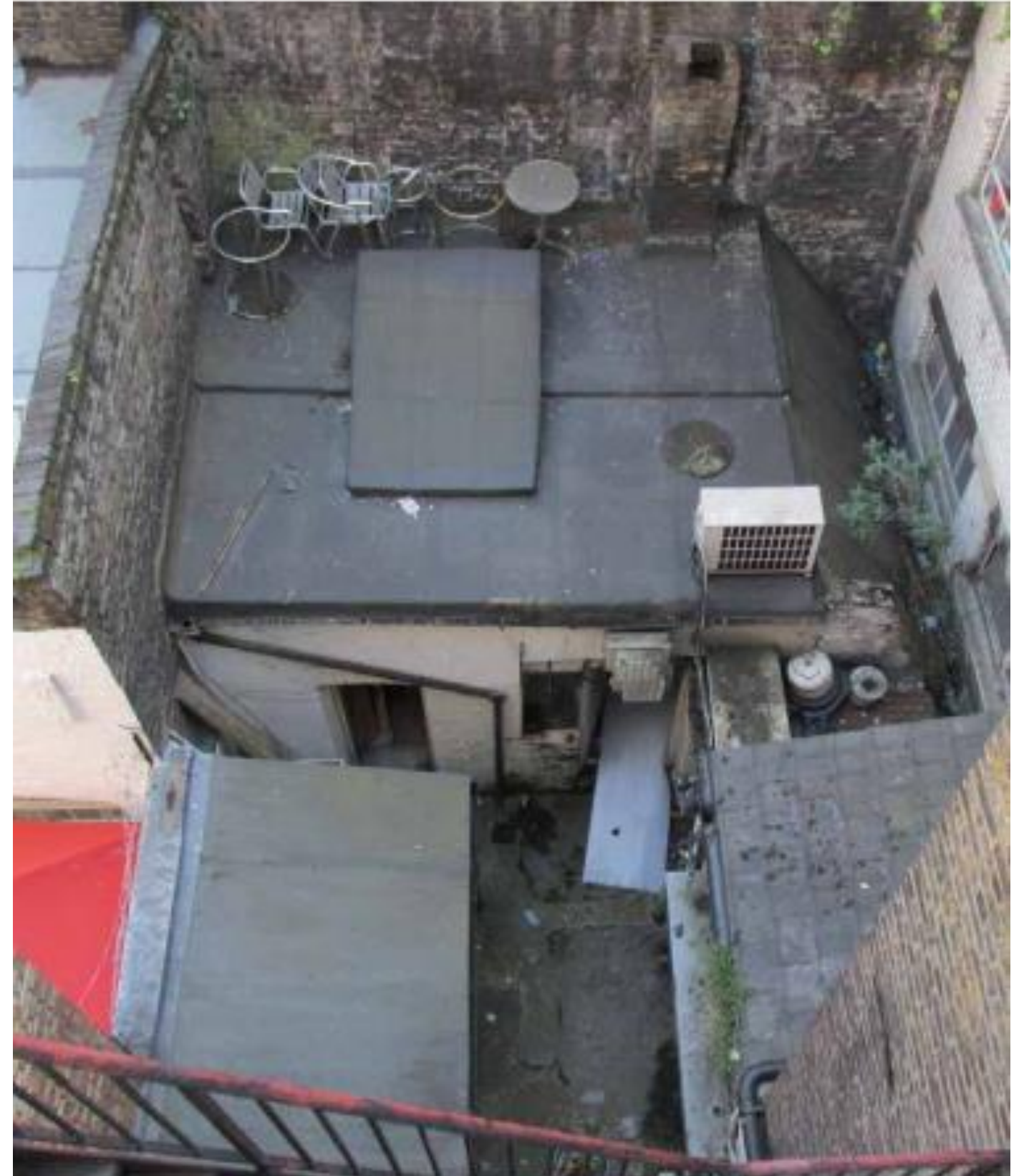
Above: View from above of rear workshop building and modern extensions
