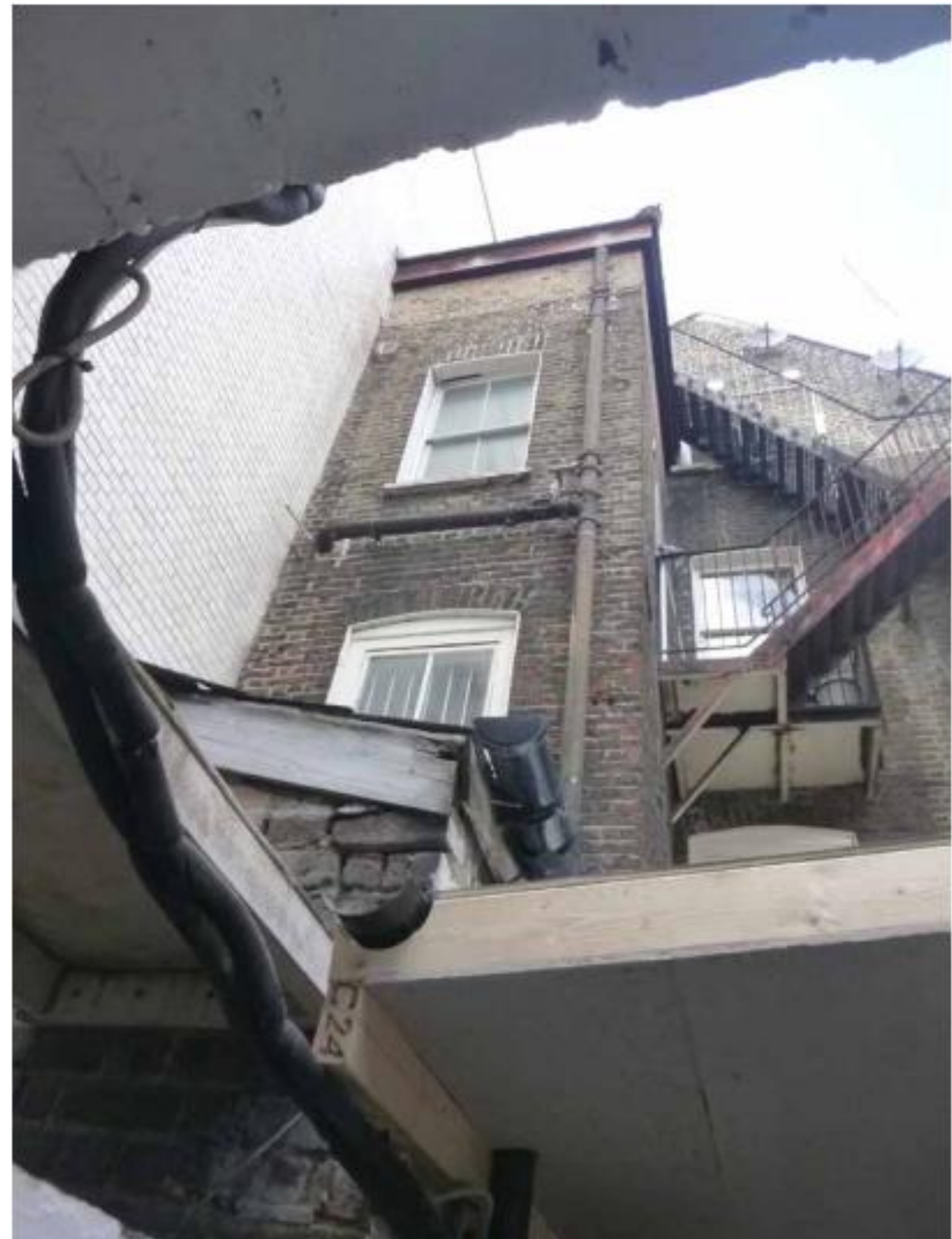
Above: Rear elevation of 7 Denmark Street, showing modern extensions
