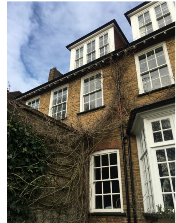
Fig. 06 - Existing rear garden
