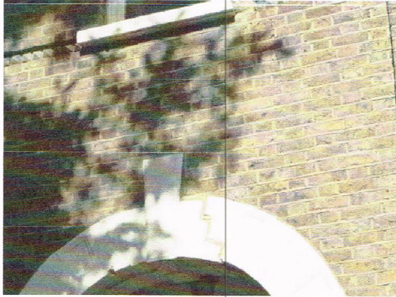
Photo 2. The cracking over the front door – further evidence of subsidence.
