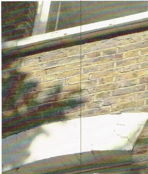
Photo 1 the diagonal crack under the top, corner window – clearly subsidence.
