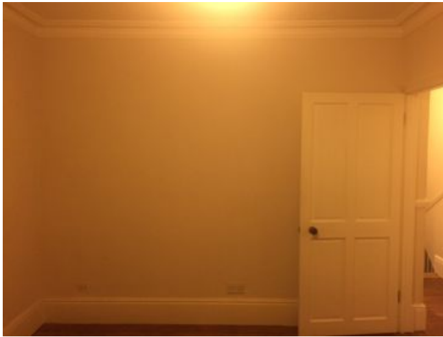
8. Ex Living room - Dividing wall to be removed as part of the open plan works and made good to match existing. Supporting nibs and downstand to be retained to form entrance between spaces.
