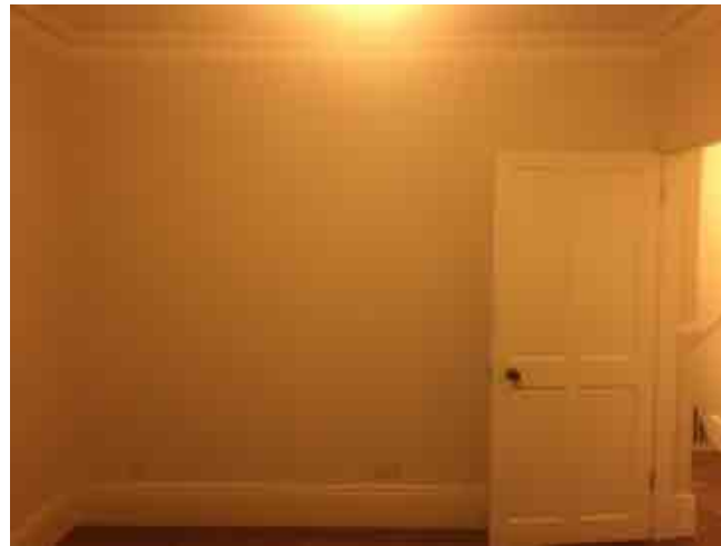
8. Ex Living room - Dividing wall to be removed as part of the open plan works and made good to match existing. Supporting nibs and downstand to be retained to form entrance between spaces.
