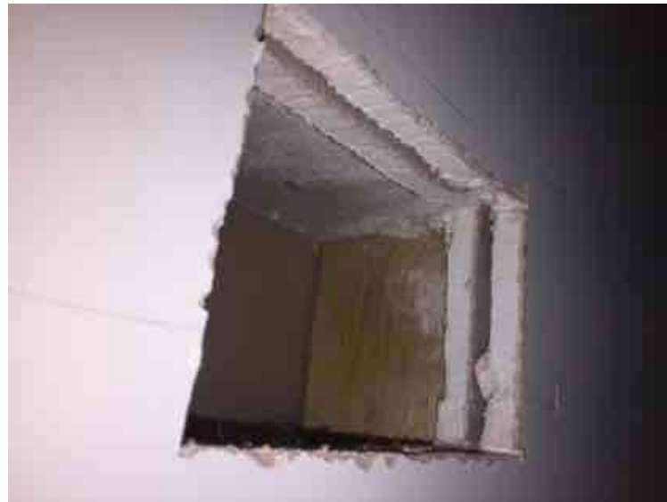
P2 - Wall construction, Plasterboard and timber frame post 1971 to wall above in Living rm, close up of timber adj
