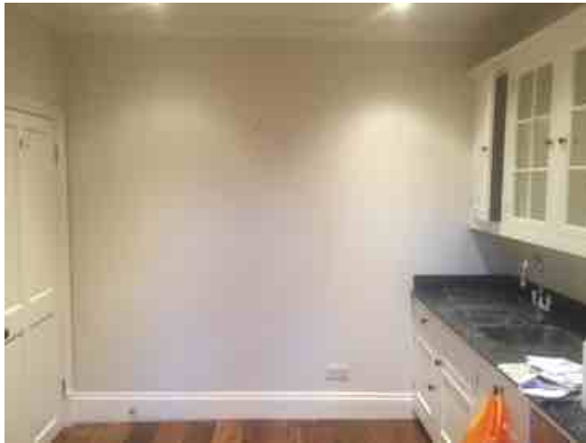
4. Kitchen (Upper ground floor) - Dividing wall between Living room and Kitchen to be removed to suit open plan design with nib walls and downstand to form opening
