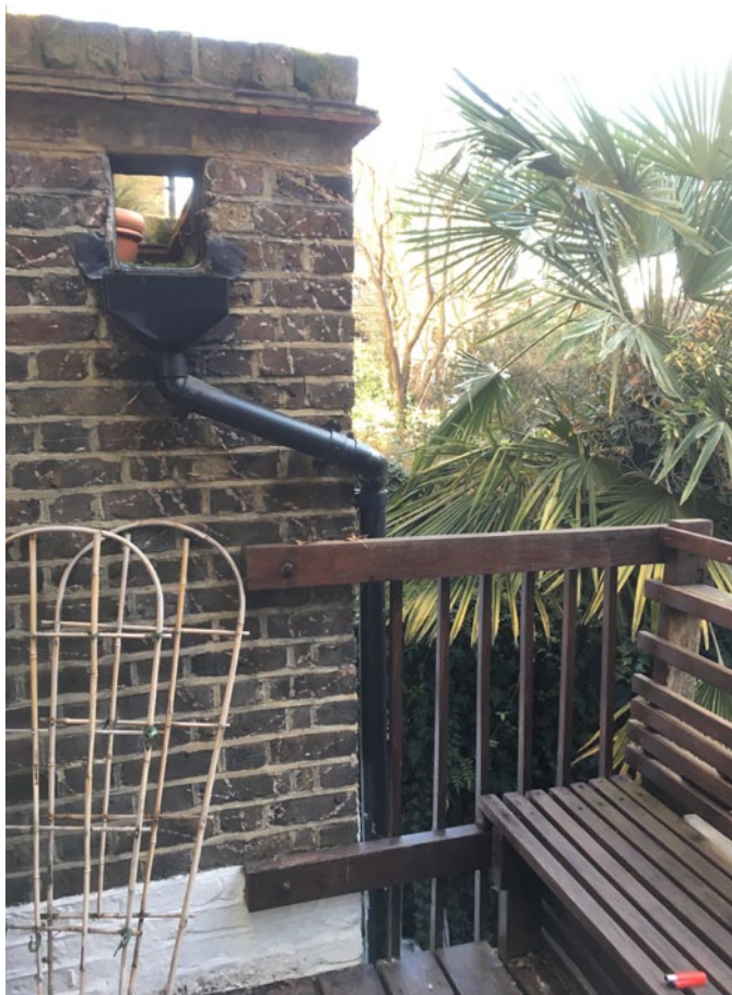
Figure 19: View of the interface between the existing balcony and original closet extension, poorly detailed.
