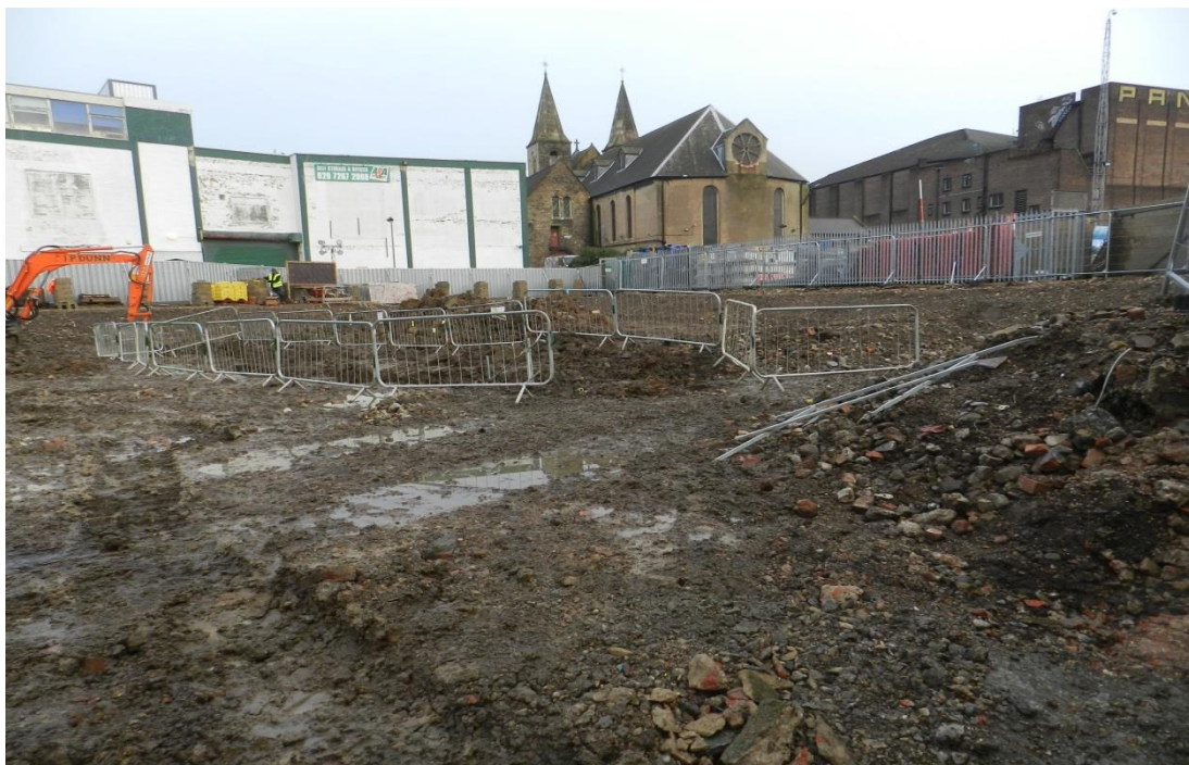
TR2 looking north-east/east towards the church of St. John the Baptist
