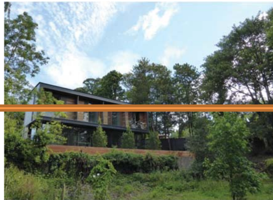
01- Neighbouring property height (rear) Orange line showing the relation of the roof of no51 Fitzroy Park with the surrounding trees. The proposed scheme is designed to match the height of no51 which is far lower than the trees surrounding the site and will not be visible from Hampstead Heath (pictured below).
