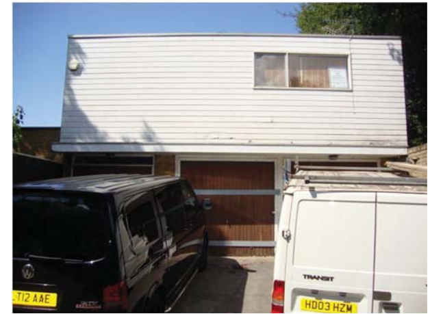
02- Existing property from Fitzroy Park
