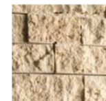
Split face/ Rigato Portland stone cladding
