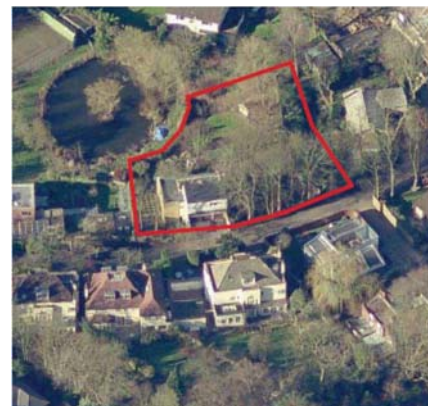
Aerial view from east
