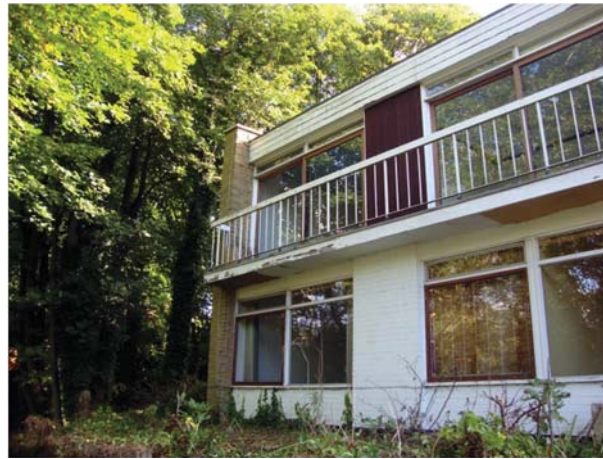
01- Existing property (rear)
