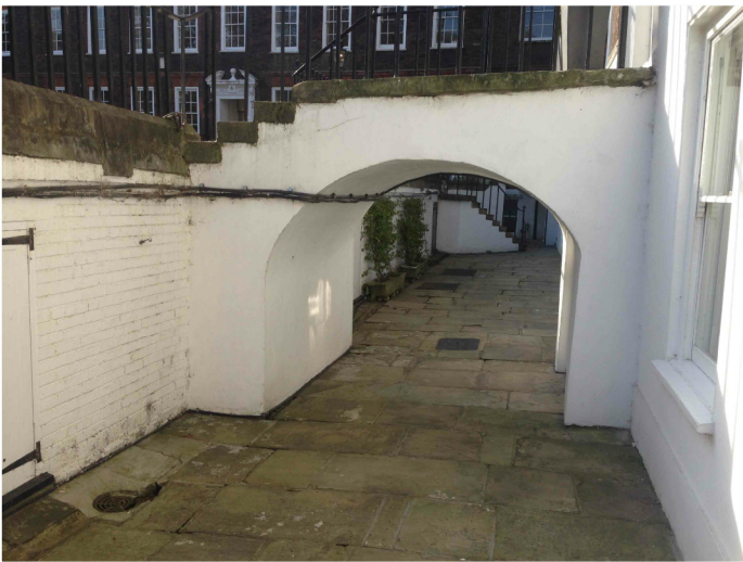
IMAGE OF EXISTING LIGHTWELL
