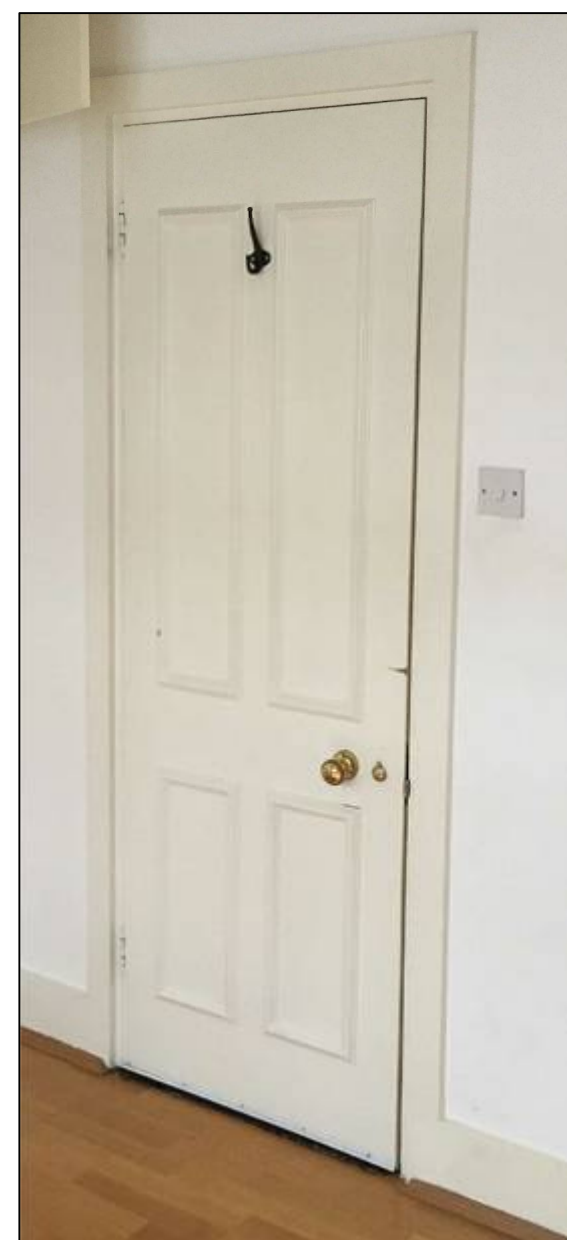
Typical Existing Door, Architrave and Skirting
