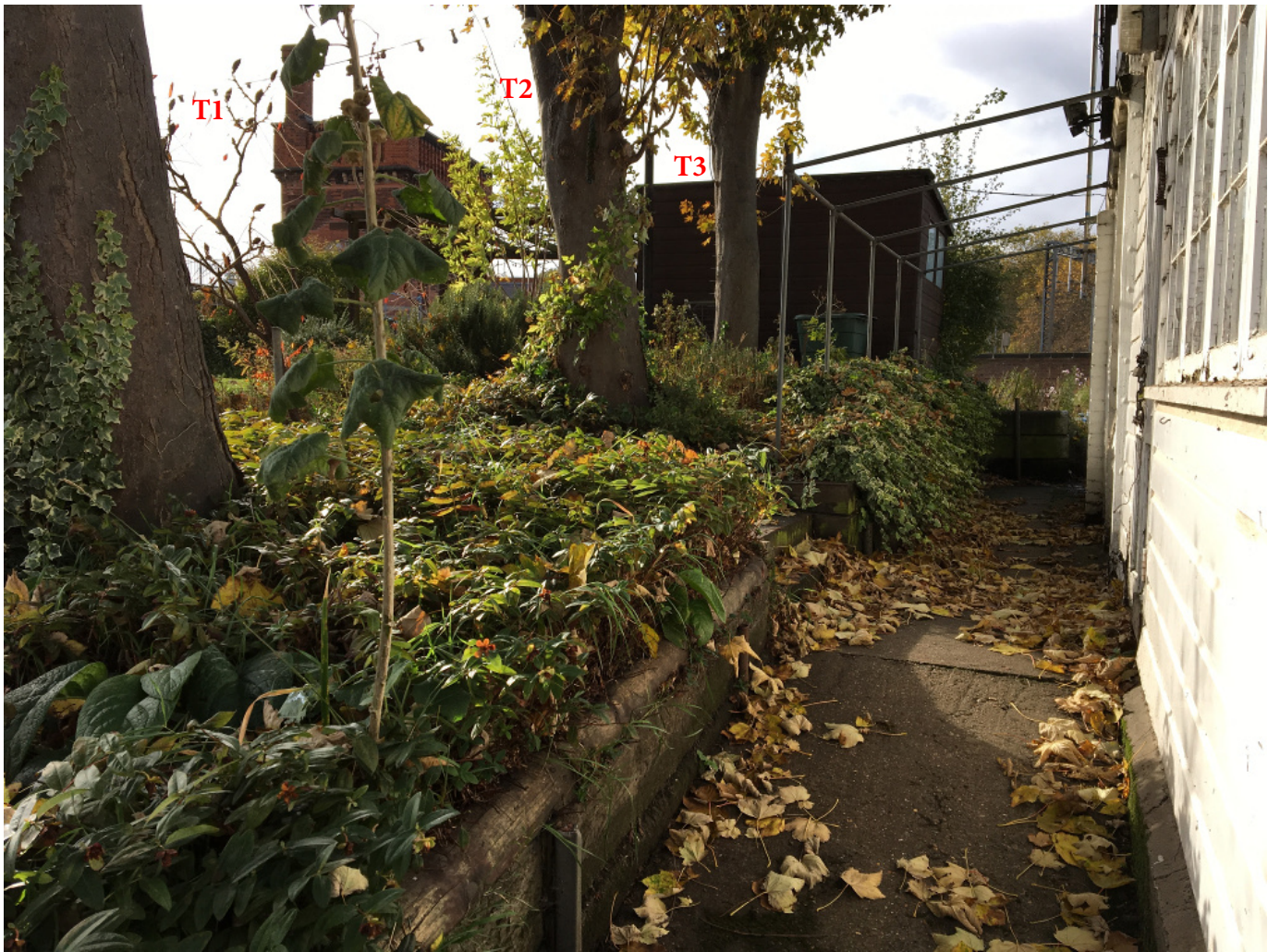
Existing path showing raised garden area with trees. Height 400mm at T1 increasing to 800mm at T3
