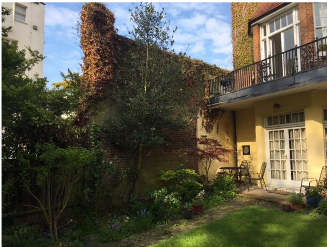
3. Boundary wall with The Coach House, Belsize Park Gardens
