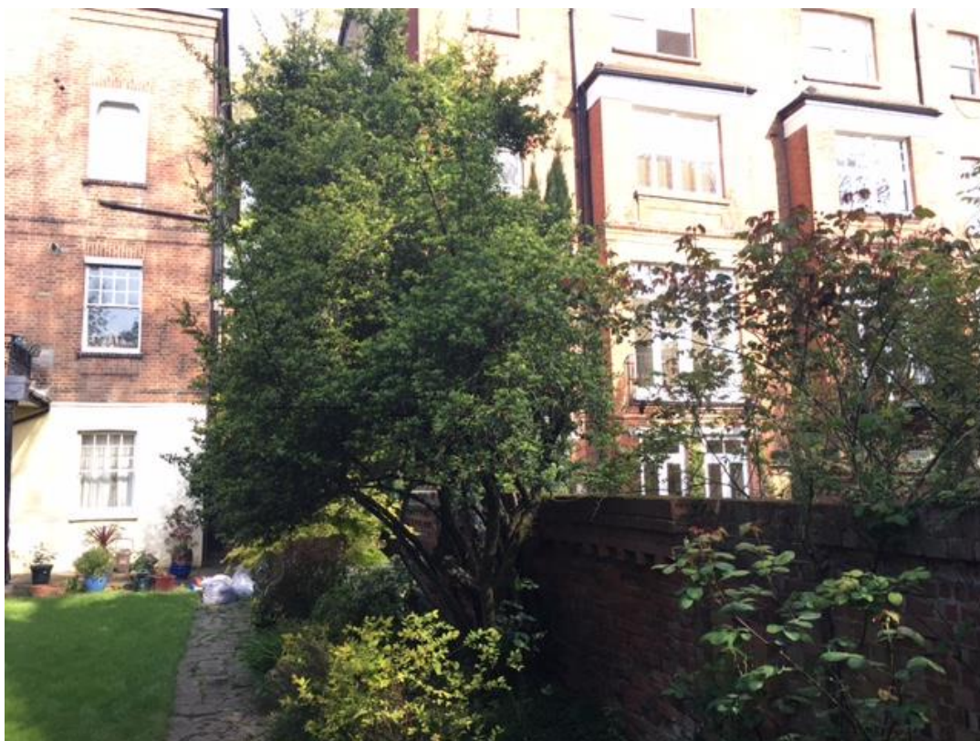
4. Rear elevation of Nos. 16 & 18
