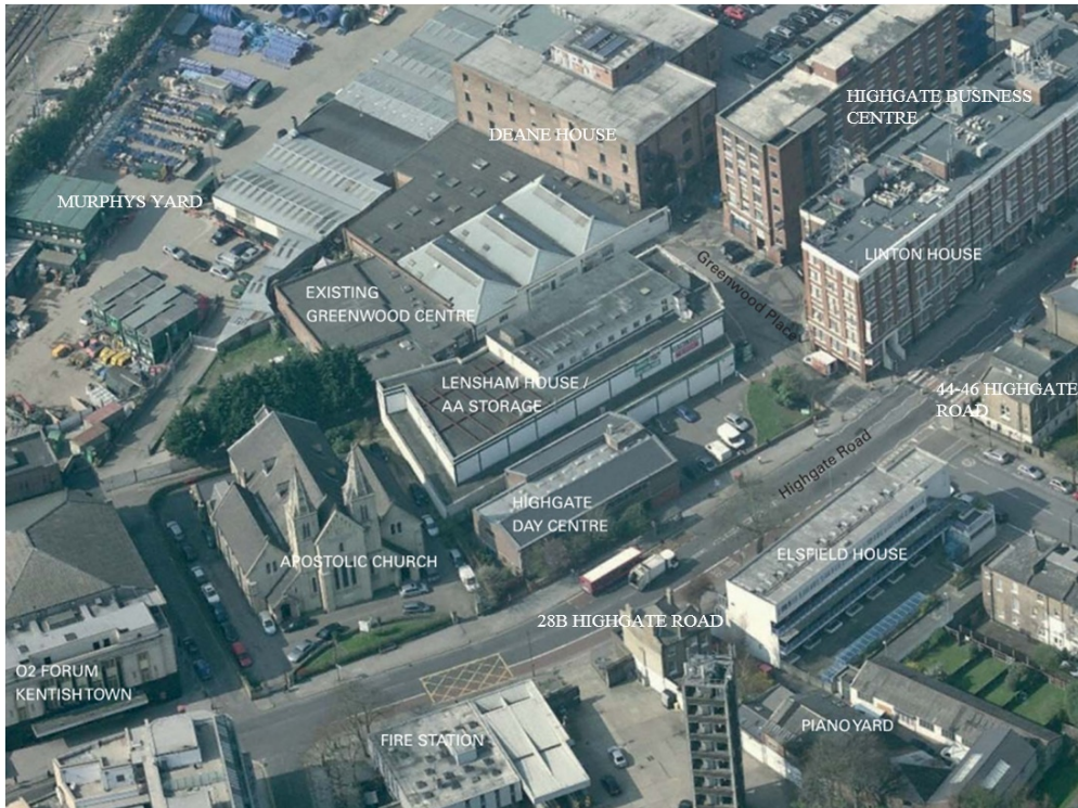
Figure 5 (above): Surrounding properties
