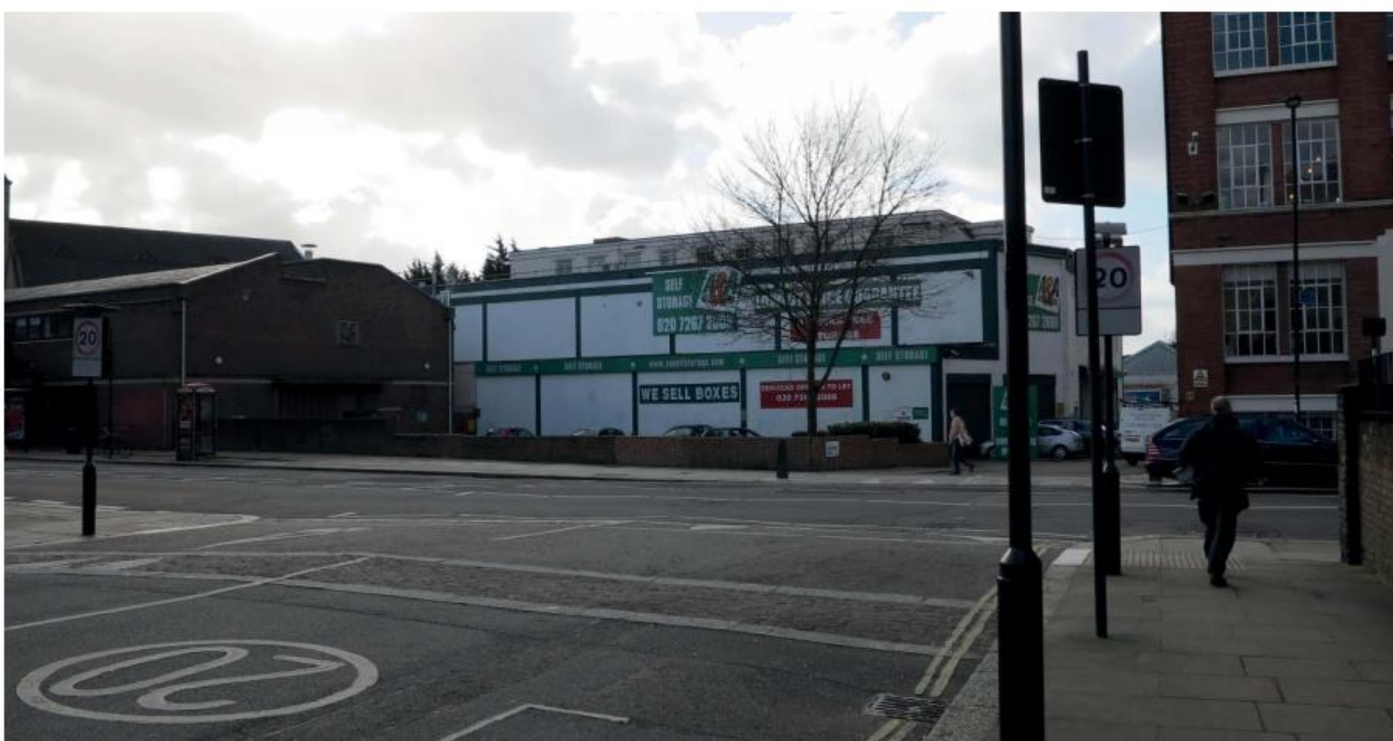
Left: Looking south over Highgate Road. A&A Self-Storage in centre of image, Highgate Centre to the left
