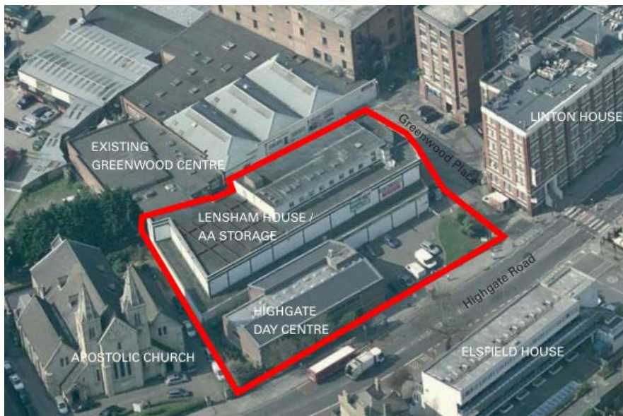
Figure 1 (above): The application site (outlined in red) including the A&A Self-Storage and Highgate Centre buildings with the Greenwood Centre to the rear, Apostolic Church to the south and Linton House to the north.
