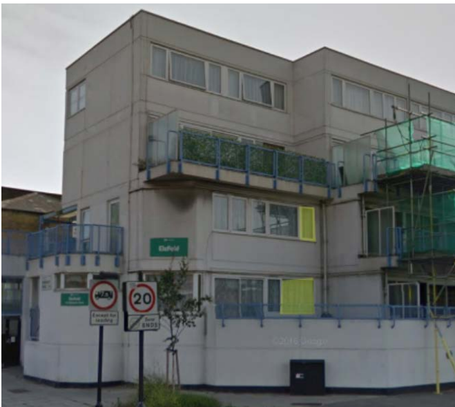
Figure 8 (left): The first floor window (highlighted in yellow) at 42 Highgate Road would retain less than 15% VSC; however, it is compromised by its position below a balcony and adjacent to a return. The rooms with a yellow highlighted window do not achieve winter APSH.
