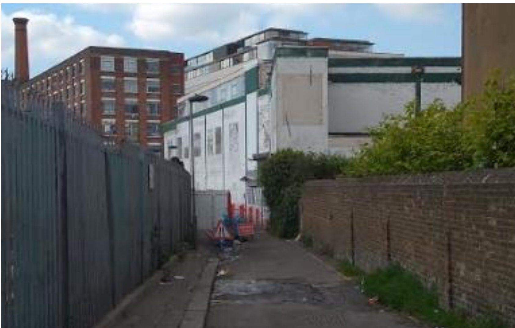
Left: Side/rear elevations of A&A Self-Storage building (centre) from Greenwood Place
