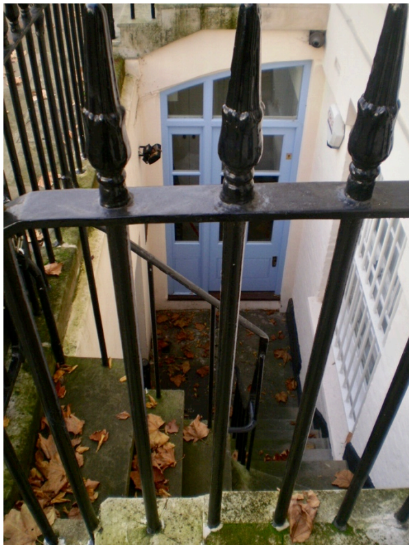
No. 19 Basement Area, Non-original door & window infill under bridge - No Significance.
