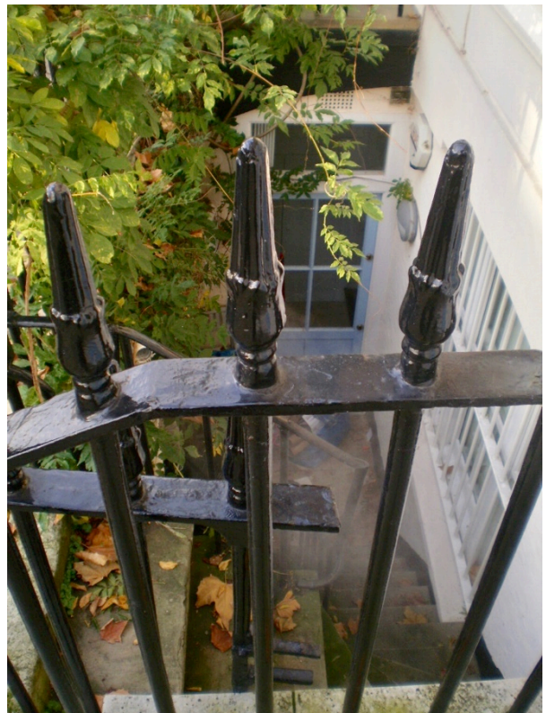
No. 20 Basement Area, Non-original door & window infill under bridge - No Significance.
