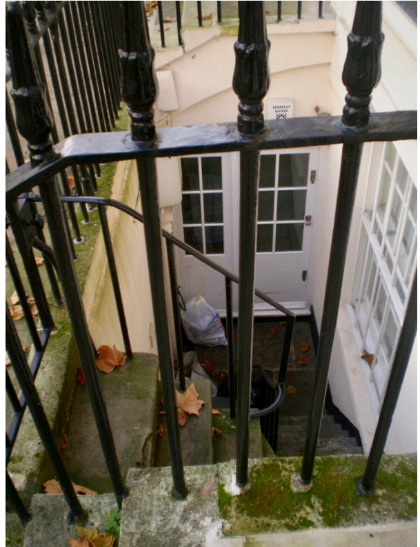
No. 18 Basement Area, Non-original door & window infill under bridge - No Significance.
