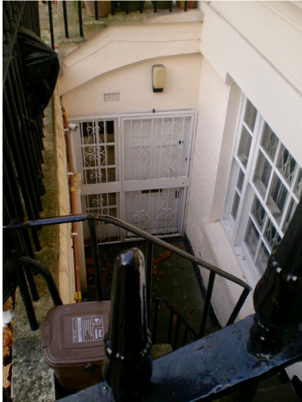
No. 21 Basement Area, Non-original door & window infill under bridge - No Significance.
