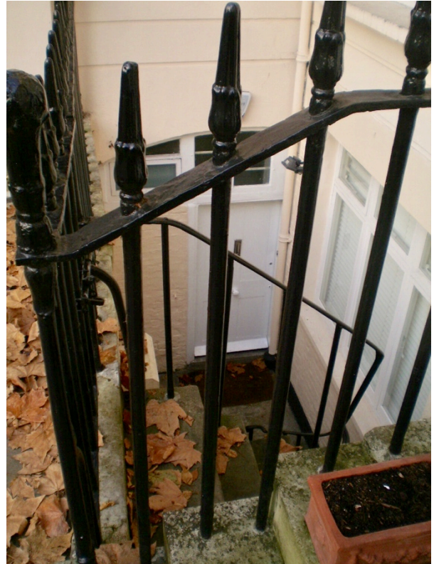
No. 22 Basement Area, Non-original door & window infill under bridge - No Significance.
