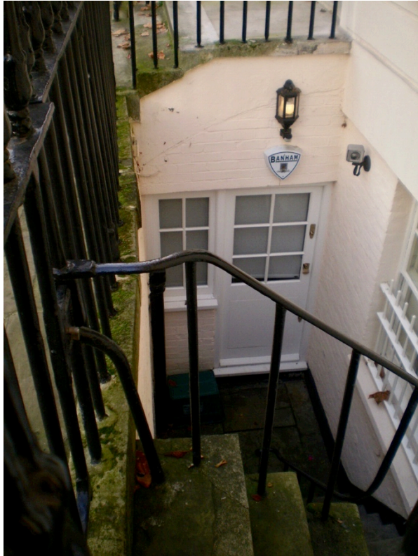
No. 17 Basement Area, Non-original door & window infill under bridge - No Significance.
