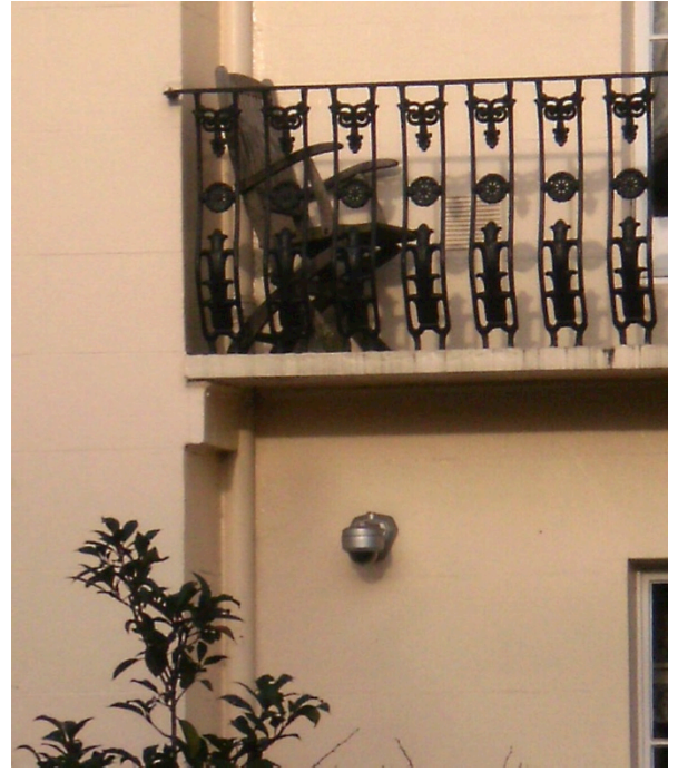
6 Prince Albert Road, Mid 19 th C detached villa. Listed Grade II. Primrose Hill Conservation Area.
