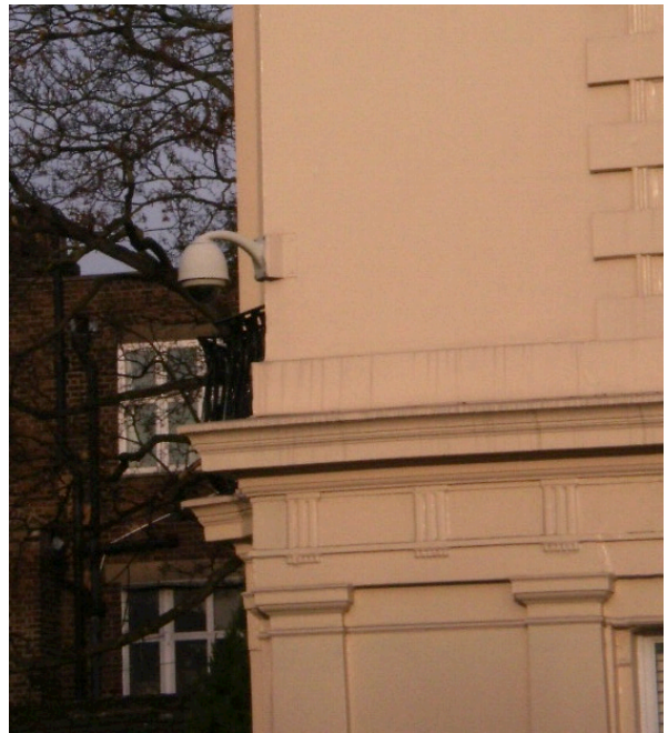
4 Prince Albert Road, Mid 19 th C detached villa. Listed Grade II. Primrose Hill Conservation Area.
