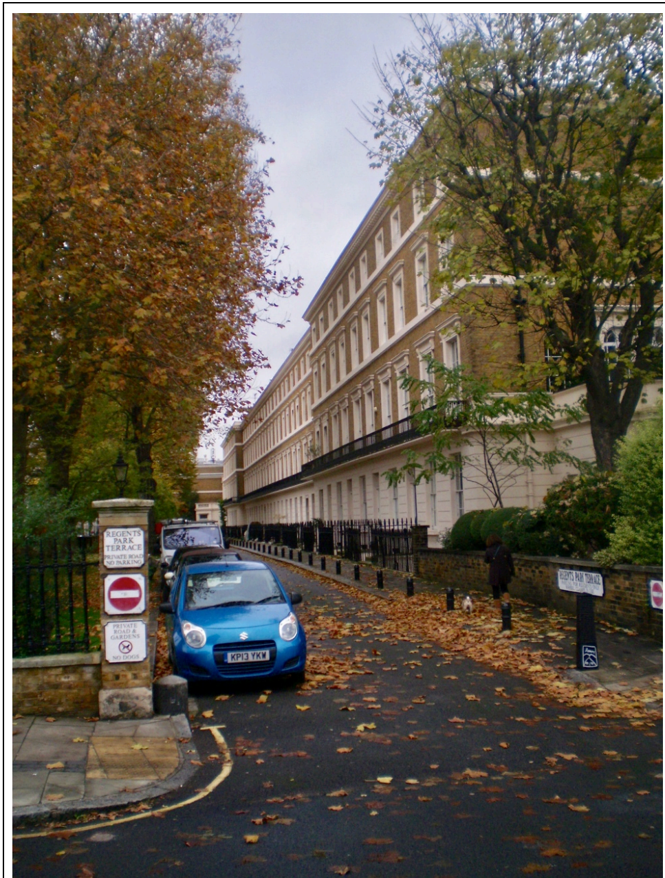
1-22 Regent's Park Terrace, view from south
