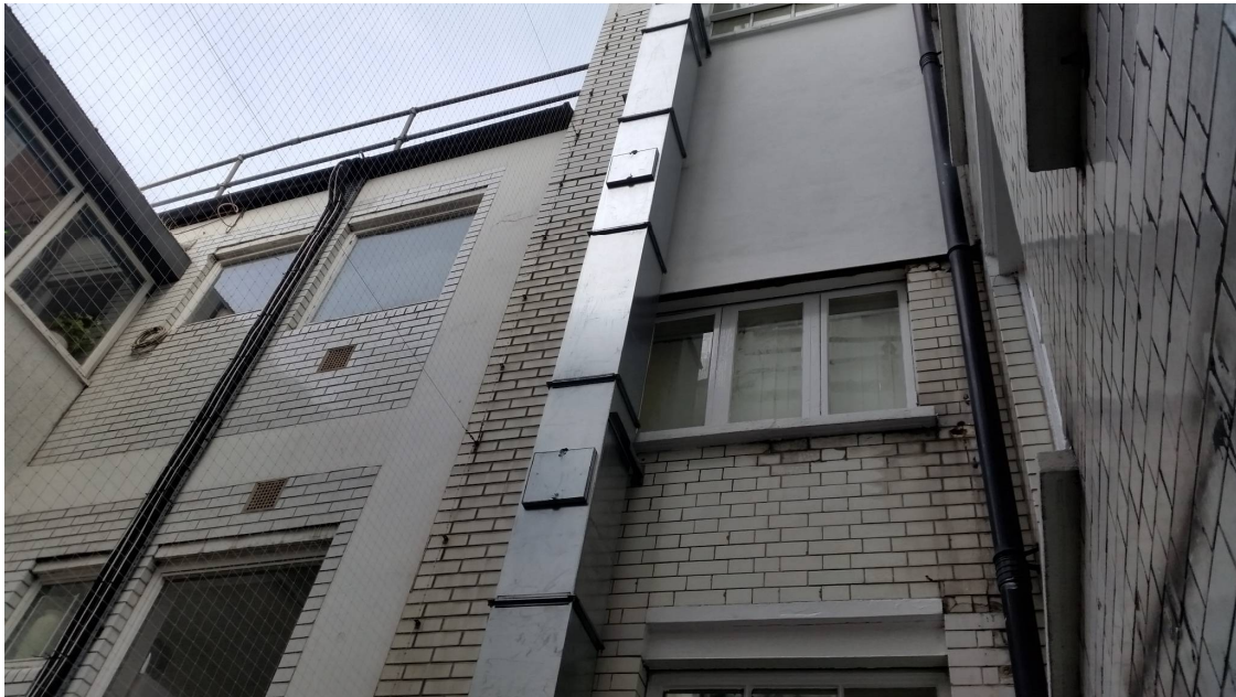
Picture 3: The extract ducting can be seen in the picture but the out let is at roof height. The picture also shows the construction of the light well.
