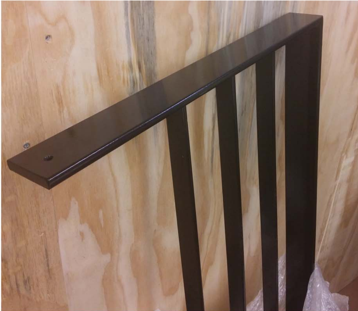
Image sample of steel balustrade delivered to site. Note balustrade will be dark grey RAL 7043 to match throughout.
