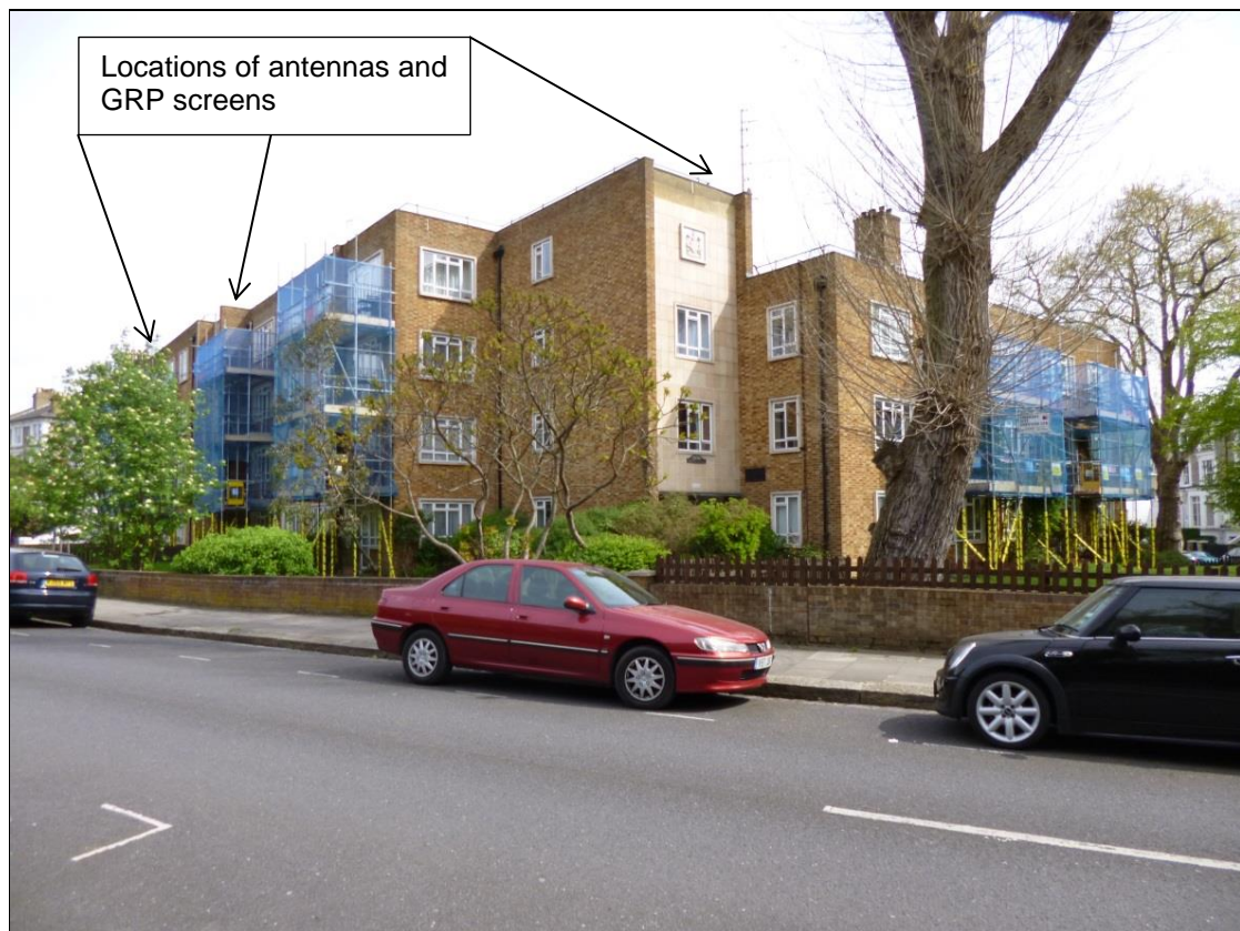
Figure 3: Troyes House, view east from west side of Lawn Road showing the corner of the L-shaped blocks - the three storey element to the right; the four storey element to the left. The 6 half-height antennas and 3 GRP screens are proposed to be sited in the northeast and southeast corners and at the front centre of the 4-storey block, to minimise the antenna height above the rooftop, with the meter cabinet against the rear elevation at ground floor level.
