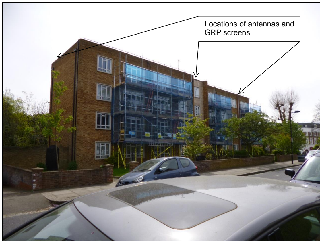
Figure 2: The appeal site view southeast from west side of Lawn Road. The 6 half-height antennas and 3 GRP screens are proposed to be sited in the northeast and southeast corners and at the front centre of the 4-storey block, to minimise the antenna height above the rooftop, with the meter cabinet against the rear elevation at ground floor level.
