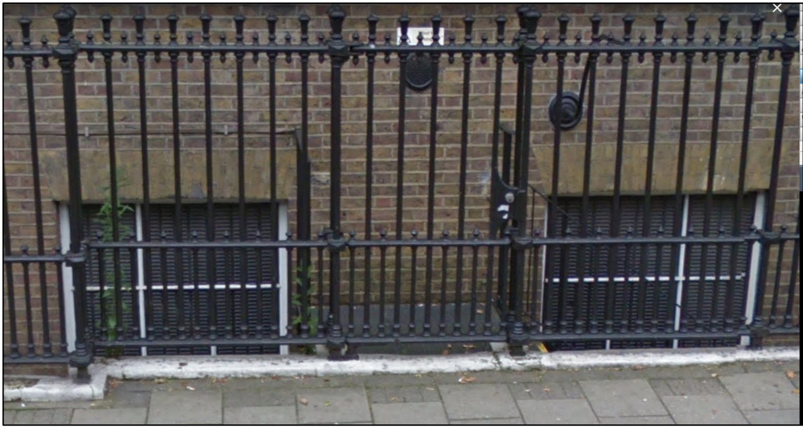
Photograph of typical basement car park window. Existing metal mesh infill panels (to be retained) obscure existing plant behind / views into car park from Eversholt St.
