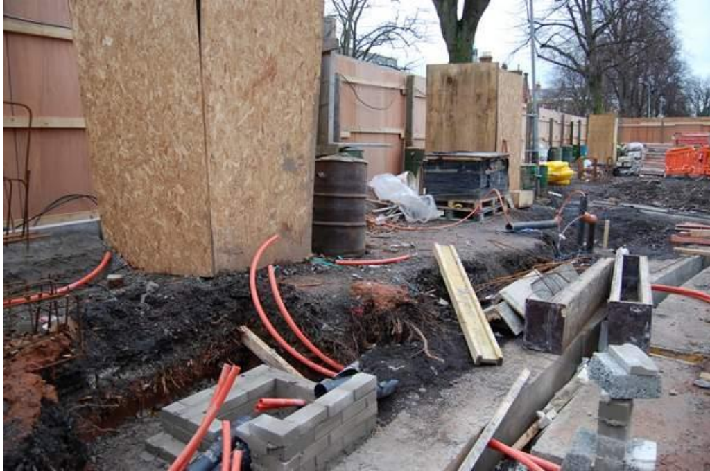
Fig 2 Example of wooden hoarding protecting tree stems from damage
