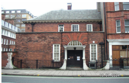
Existing front entrance
