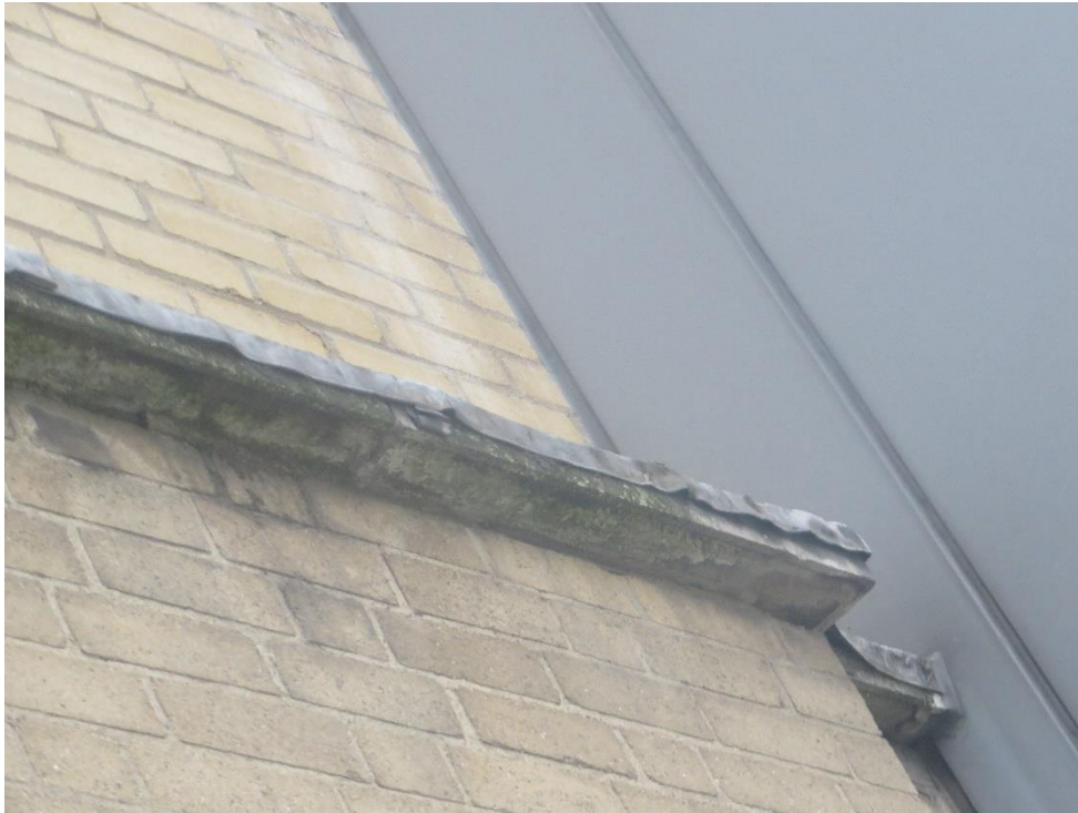
Minor lifted flashing viewed from the 2 nd floor front roof top
