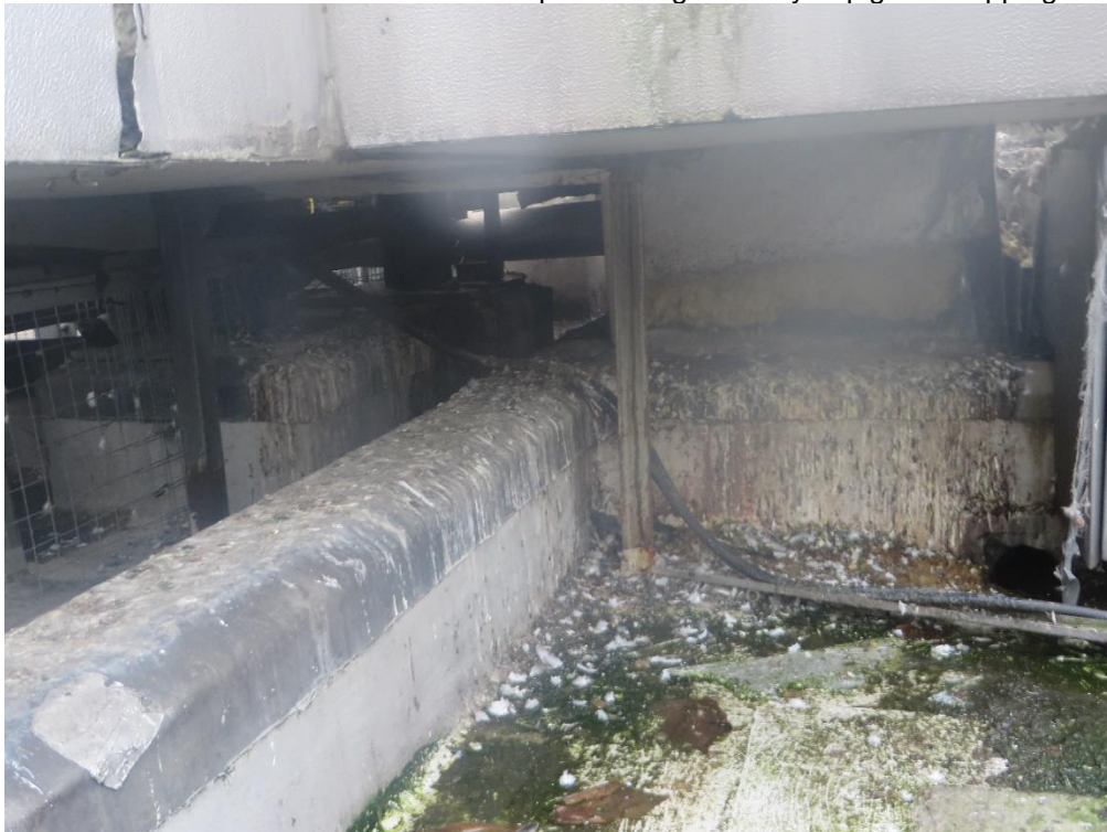
The sheltered area on the 6 th floor roof top with a high density of pigeon droppings and feathers
