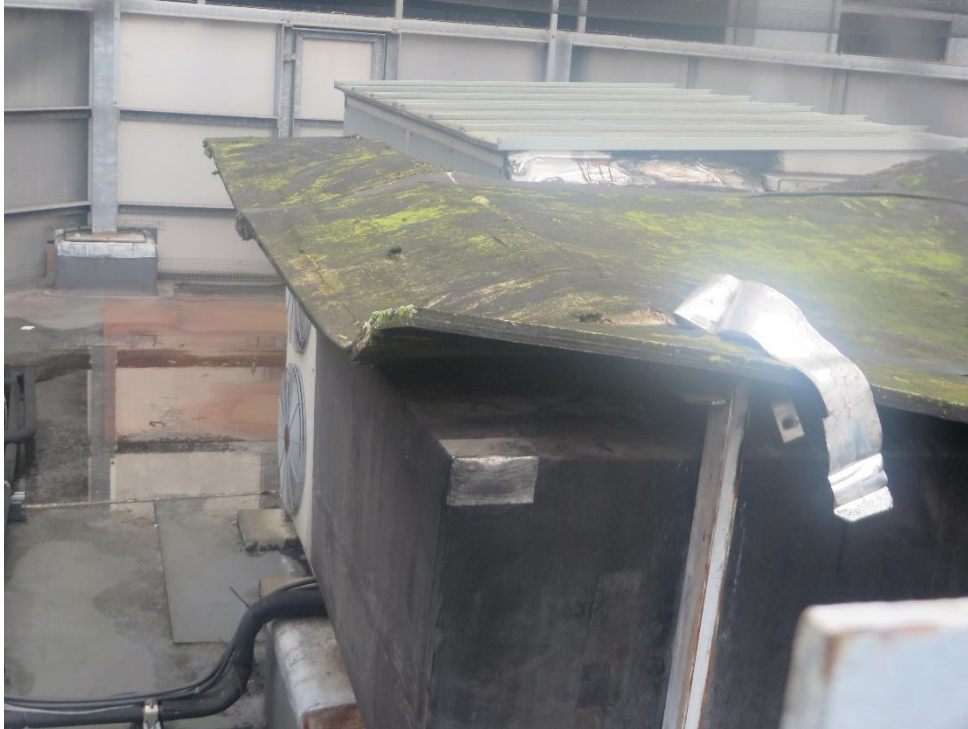
The degraded plant roof on the 2 nd floor roof top
