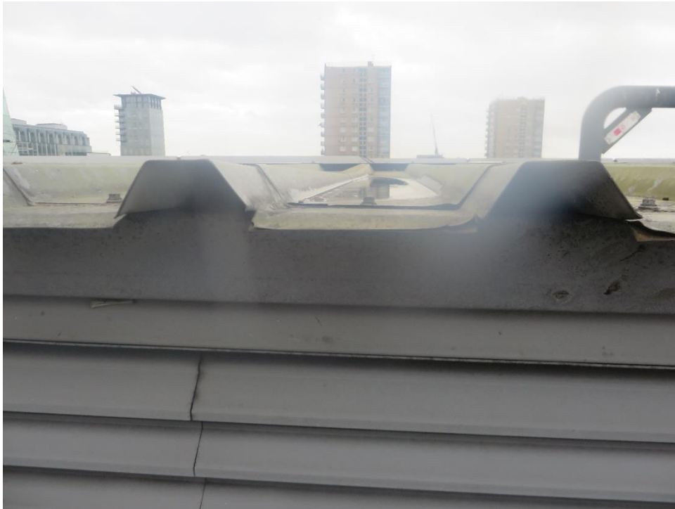
The gaps underneath the corrugated metal roof of an extractor unit
