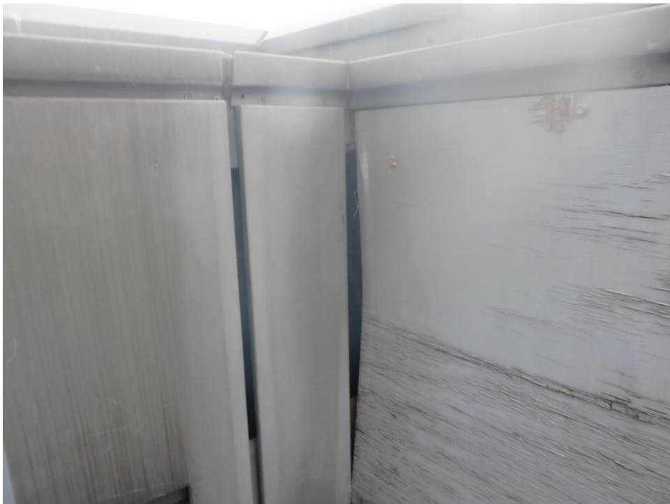
The gaps in metal hoarding encountered across most of the roof tops of B1
