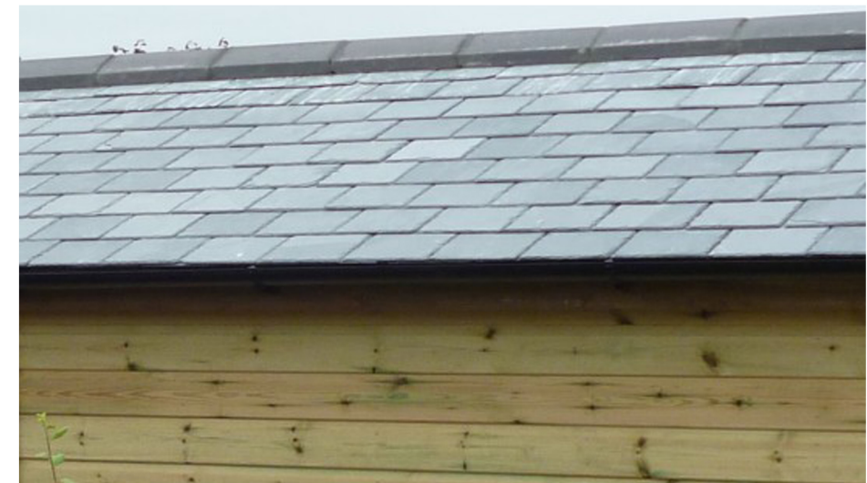
Example of slate roof on garden building
