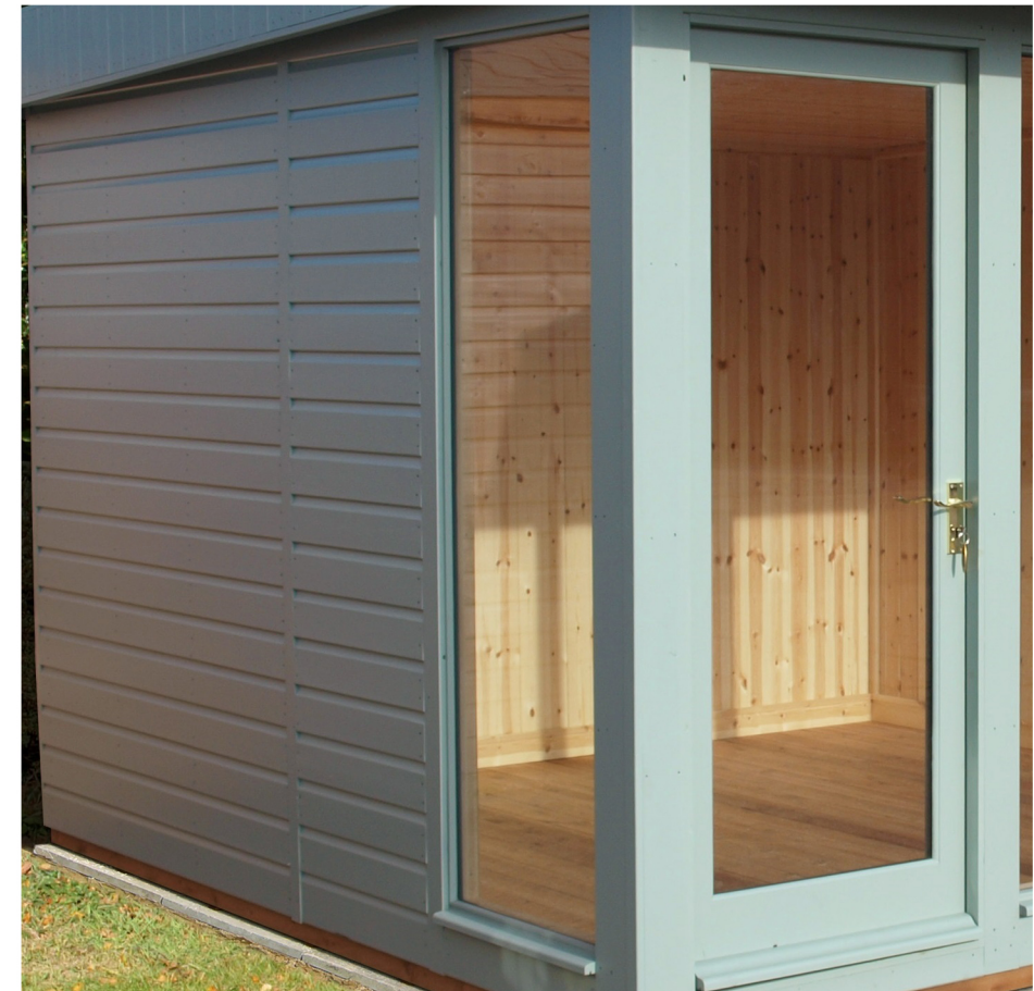
Example of pre-painted timber cladding (matt eggshell finish)
