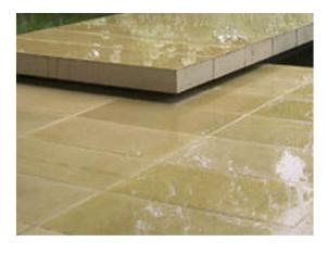
DRAINAGE Discreet slot drain solution to paving
