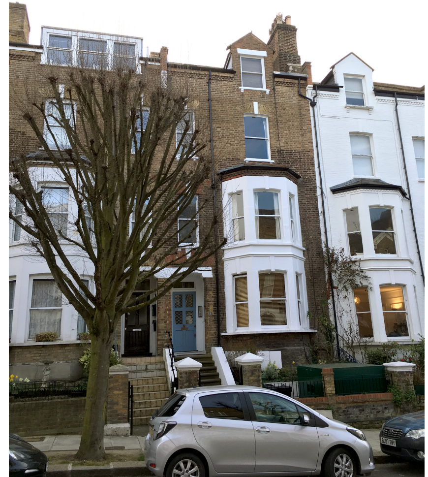
Figure 1. No 5 South Hill Park, 2017.
