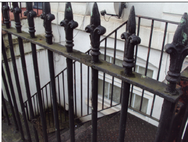
Figure 3 Railings to Lightwell
