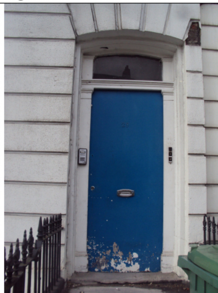
Figure 4 View of Front Door
