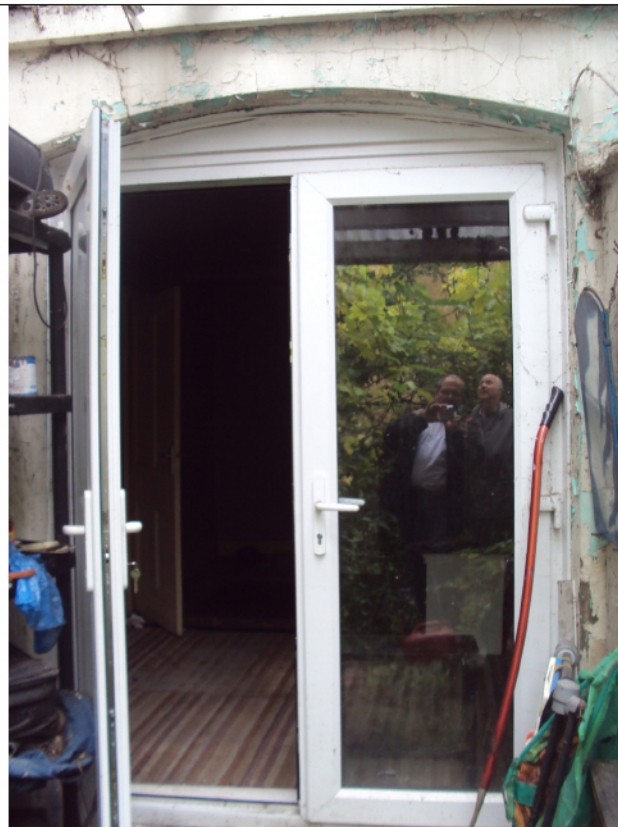
Figure 6 French Doors to Lower Ground Floor
