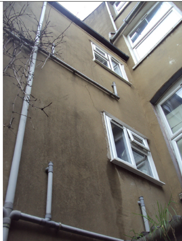
Figure 5 Rear of Property
