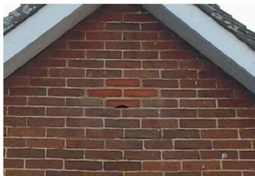
Bat box internal view, and Bat box fitted in brick with access hole at base. Brickwork shall be as per specification covered in Condition 4.
