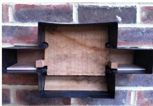
Bat box internal view, and Bat box fitted in brick with access hole at base. Brickwork shall be as per specification covered in Condition 4.
