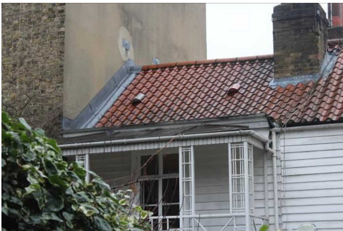
31. The balcony roof can be seen here to be zinc or lead, further investigation recommended.
