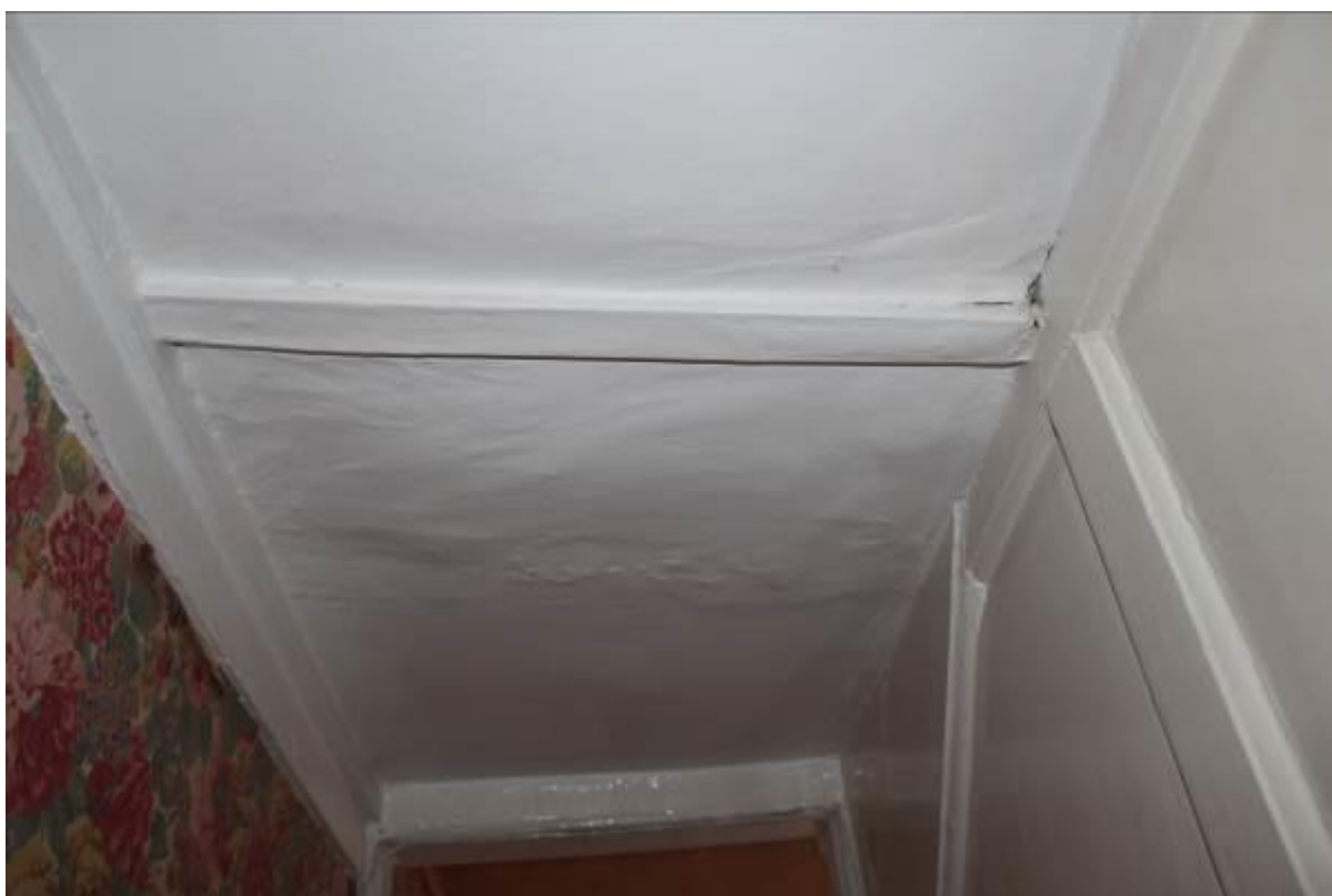
37. Overboarding recommended to first floor ceilings
