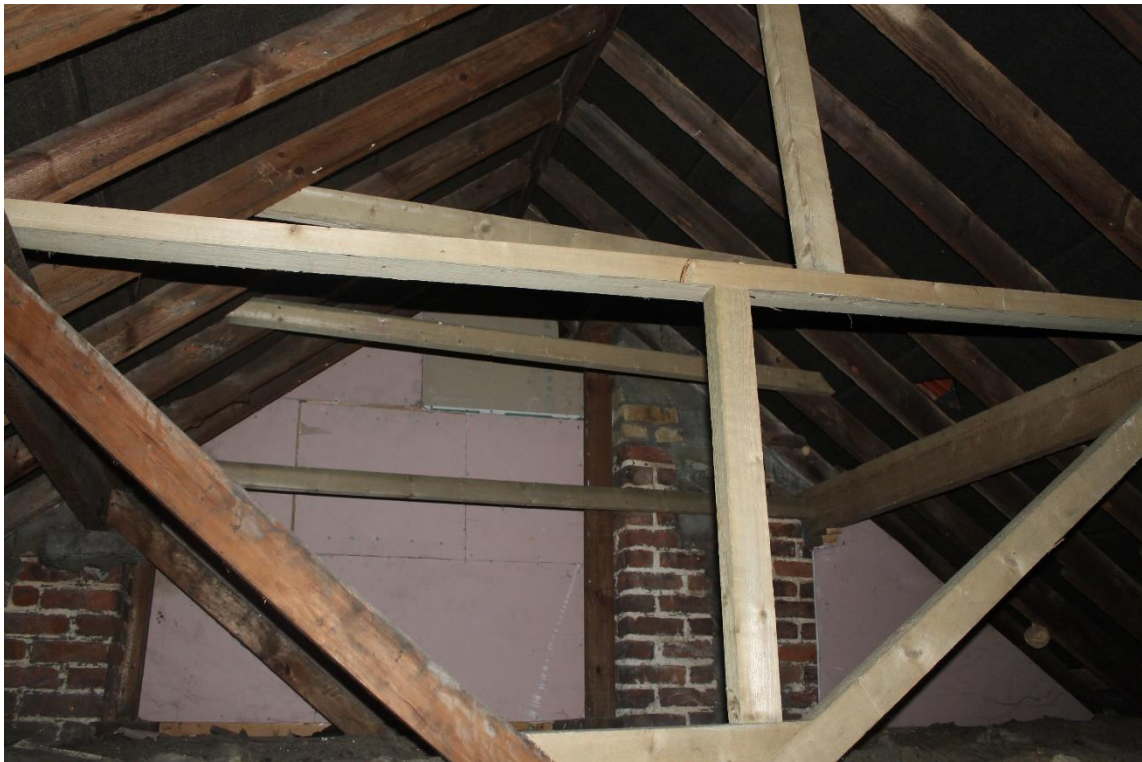
Fig.12 The roof space of the main house, looking south
