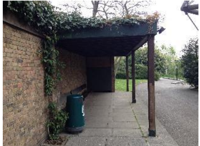
Photograph 4. Shelters to the north side of the aviary.
